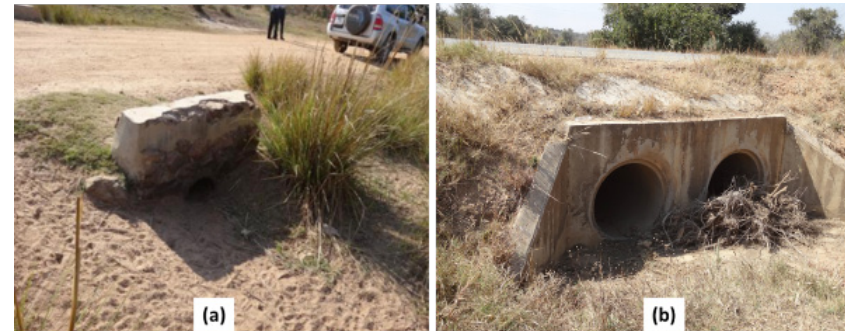
Figure 8. Silting-up/blockages of culverts in Zambia: (a) a pipe culvert blocked with sand and silt, and (b) a pipe culvert blocked with woody debris
