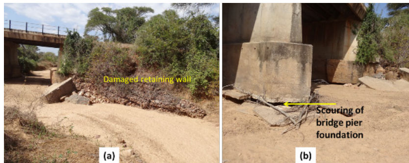
Figure 10. Water-related effects on bridges in Zambia: (a) damage to retaining walls, and (b) scouring of bridge pier foundations
