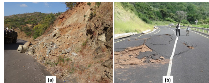
Figure 12. Slope failures in Zambia: (a) debris slides that block roadside drains and result in frequent maintenance (photo: MetaMeta), and (b) road damage due to a large-scale slide (Photo: RDA: http://www.rda.org.zm/index.php/news/278-section-of-luangwa-feira-road-damaged )
