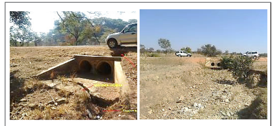
Figure 9. Examples of erosion downstream of culverts in Zambia
