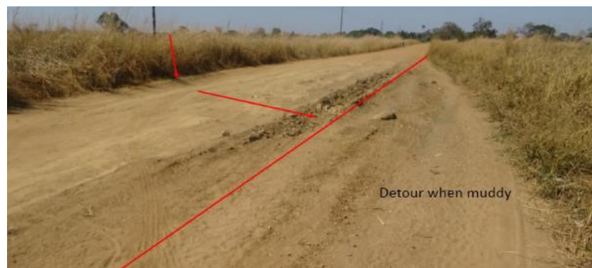
Figure 13. Loose road surface on a WB-funded, low-volume road; developed as a result of the absence proper drainage structures
