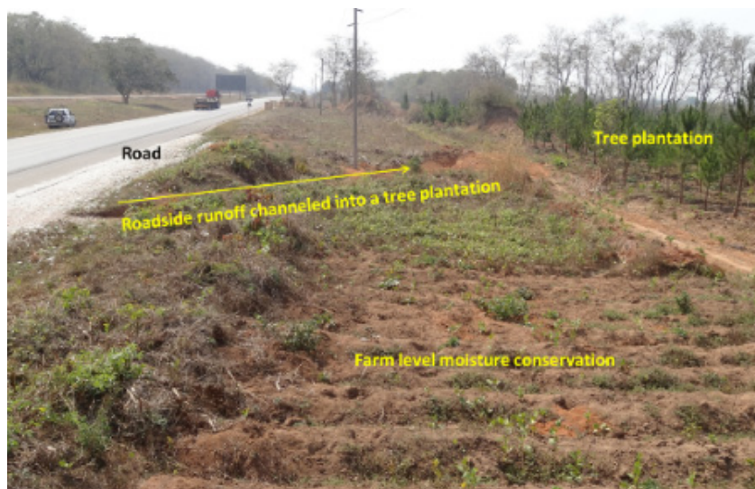
Figure 16. Water from roadsides diverted to tree plantations in Zambia
