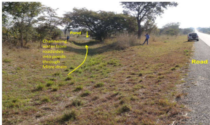
Figure 14a. Borrow pits used to store road water using mitre drains in Zambia
