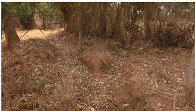
Figure 3: Diversion before the road runoff enters the farm
