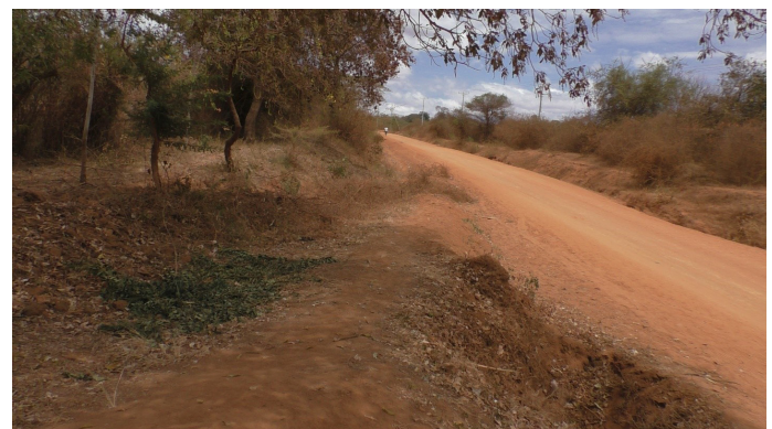
Figure 1: The road catchment towards Mwanias farm is steep and long (over half a kilometer) and therefore water flows very fast in the side drains
