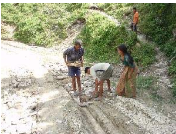
Repairing ruts and potholes
