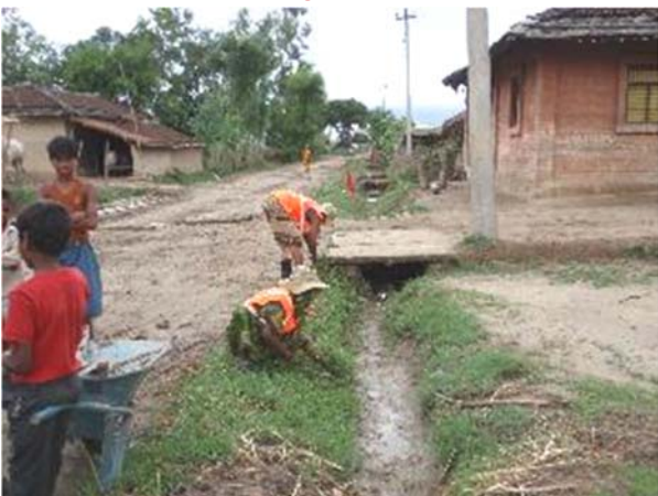
Clearing and cutting vegetation
