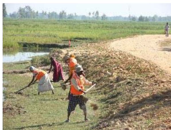
Repairing the road shoulder
