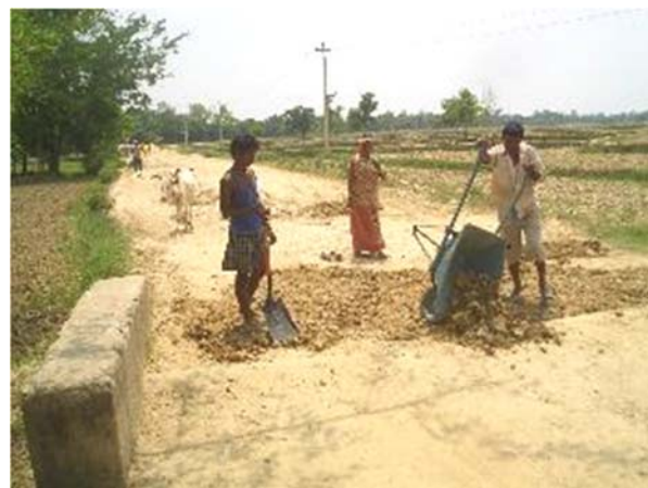
Repairing the backfill over culverts
