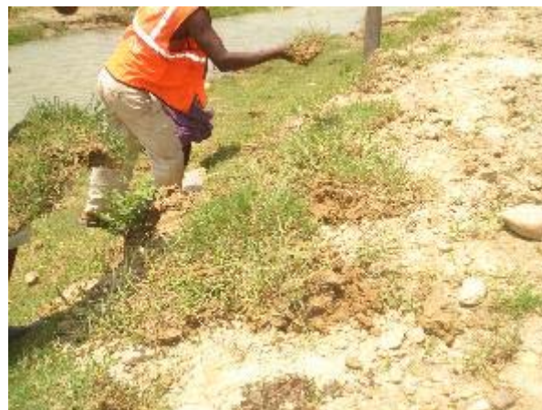
Protection of slopes by planting vegetation
