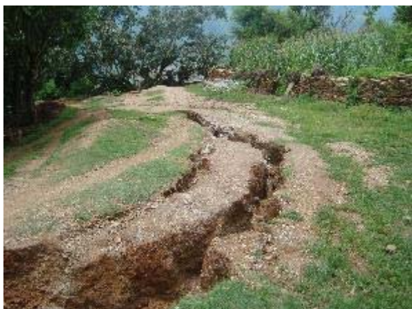
Erosion of the road surface
