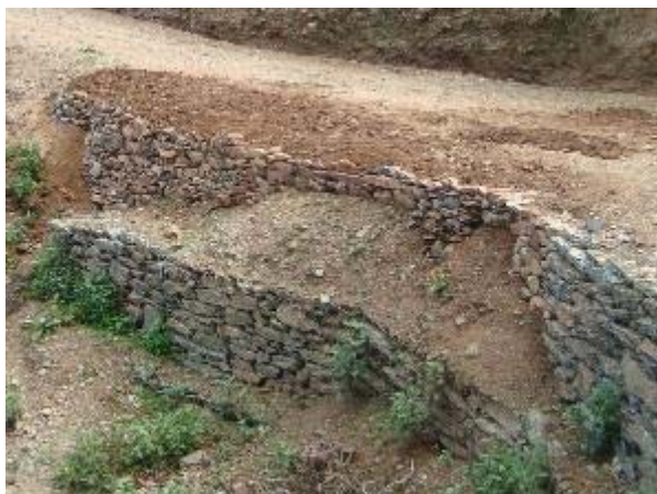
Creation of dry stone retaining walls
