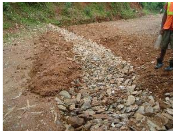
Creation of stone paved water crossings
