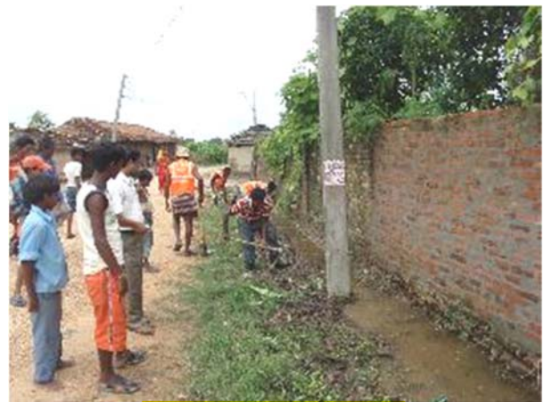
Clearing drainage ditches
