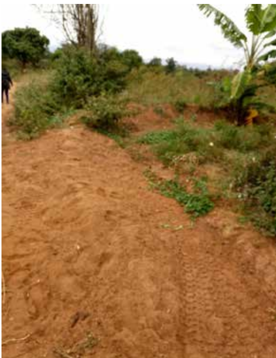
Figure 14: A cutoff drain that divert and convey road runoff into Mrs. Eunice's farm
