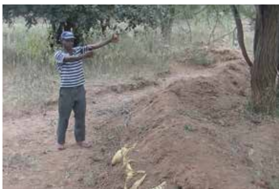
Figure 8: Mr. Mutia illustrating how the road runoff is diverted into his farm
