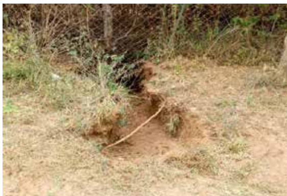
Figure 7: A cutoff to divert road water either directly into the farm or storage (farm pond)
