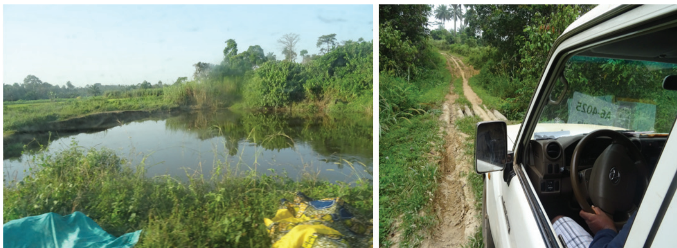
Figure 3: Roads in Foya (a) Impoundment created as a result of low volume roads construction (b) roads with no significant impacts but not accessible during rainy seasons
