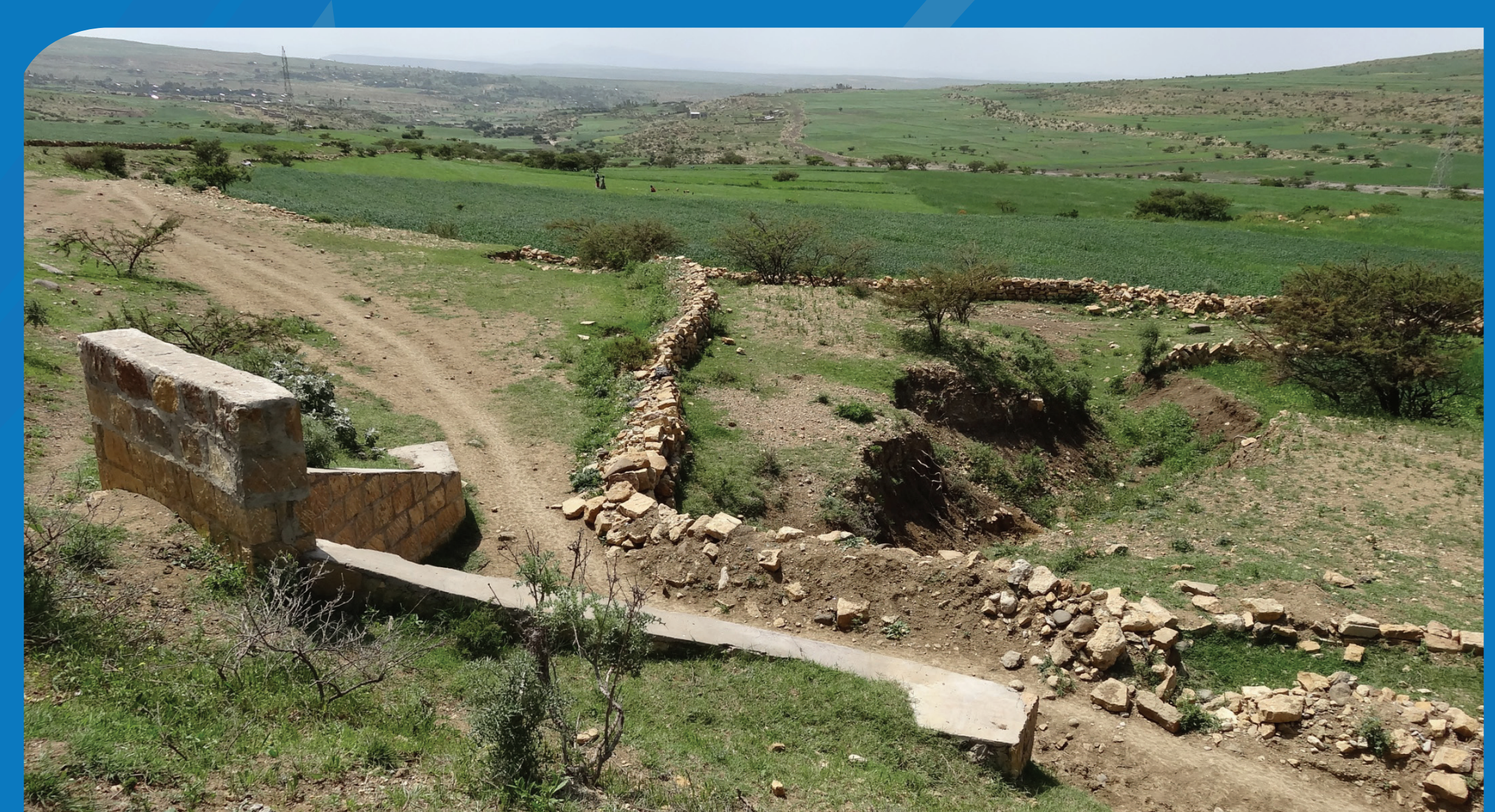
Water from a culvert directed and spread into farmlands
