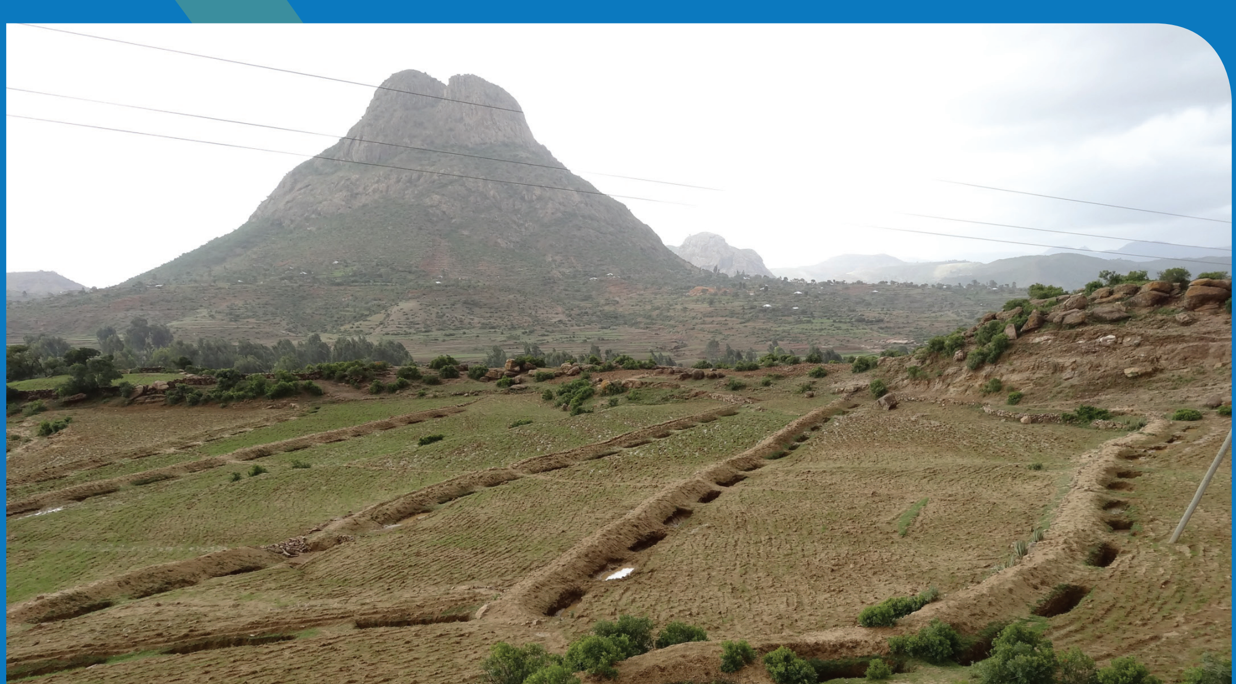
Deep trenches at downstream side of roads used to recharge groundwater
