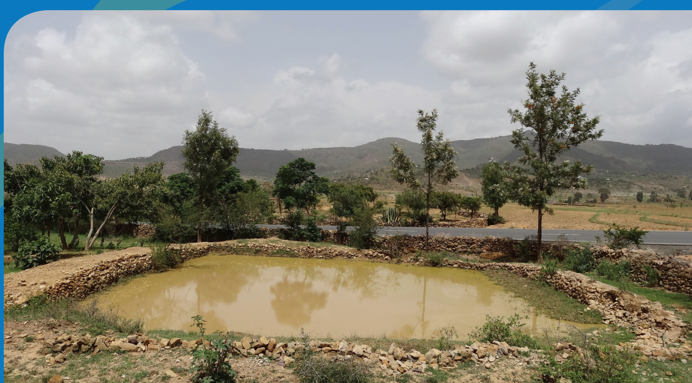
Road side run-off diverted into ponds
