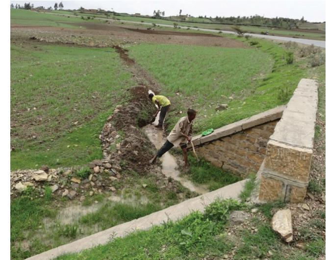
Flood water spreaders from road surface to enhance soil moisture and recharge groundwater
