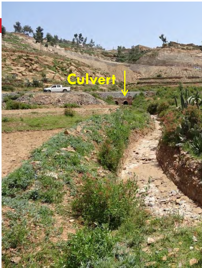
Panoramic view of channels to divert water from culverts into a borrow pit shown in (g).
