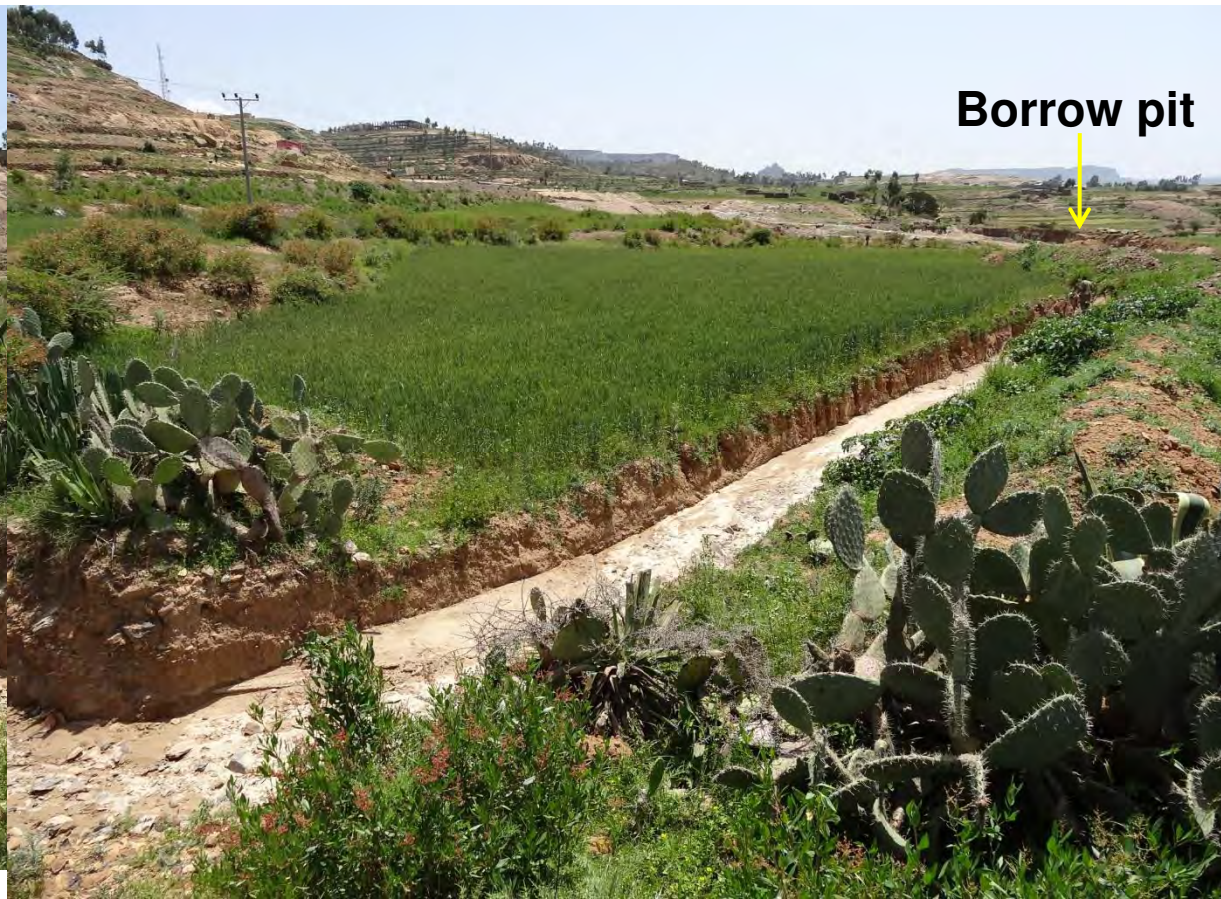
Panoramic view of channels to divert water from culverts into a borrow pit shown in (g).
