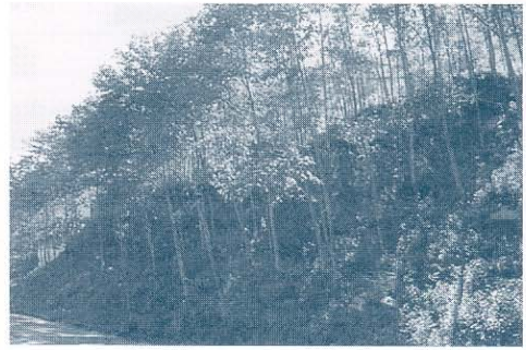
This eight-year old utis plantation, raised from polypot seedlings, is established enough to reinforce and anchor the roadside slope
