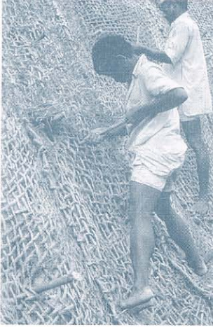
Ensure that the jute netting is loose enough to be held against the surface over the whole slope (left). Live pegs will grow to add more strength to the slope
