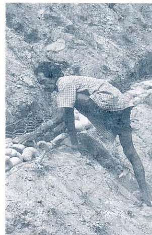
Constructing a wire bolster (see construction step 5, overleaf)
