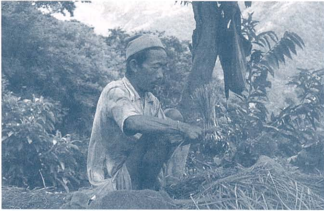
Grass slips must be prepared carefully for use on site
