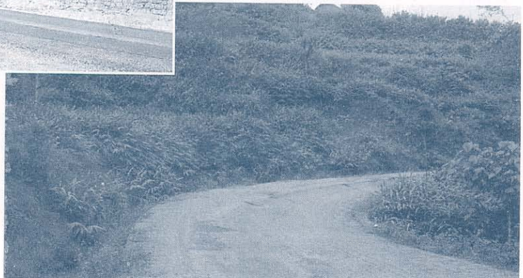
A recently rehabilitated road pavement (above): its longevity depends on the protection and maintenance of the adjoining slopes. Well-maintained roadside slopes (right). The vegetation is managed and cut on a regular basis
