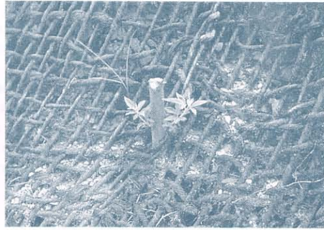
Ensure that the jute netting is loose enough to be held against the surface over the whole slope (left). Live pegs will grow to add more strength to the slope
