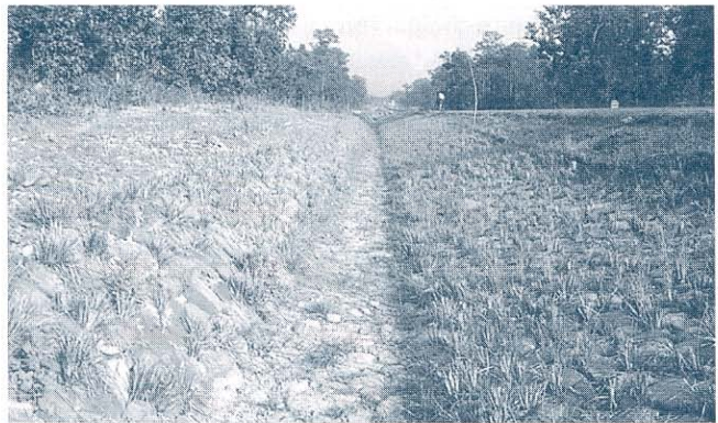
Cobbling with vegetation planted between the stones provides strong armouring
