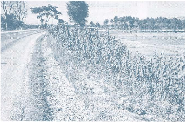
Turfing provides instant surface protection, as used on this road shoulder (the embankment has been treated with grass lines and brush layering)
