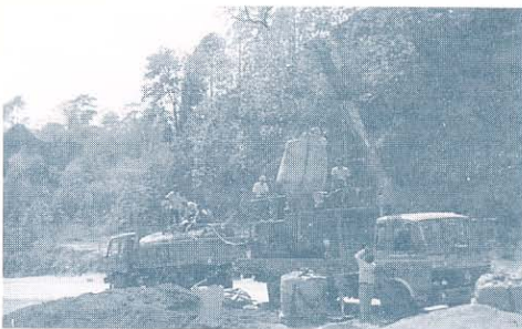
Manual methods of bio-engineering are cheaper and easier to implement than mechanical techniques such as hydro-seeding
