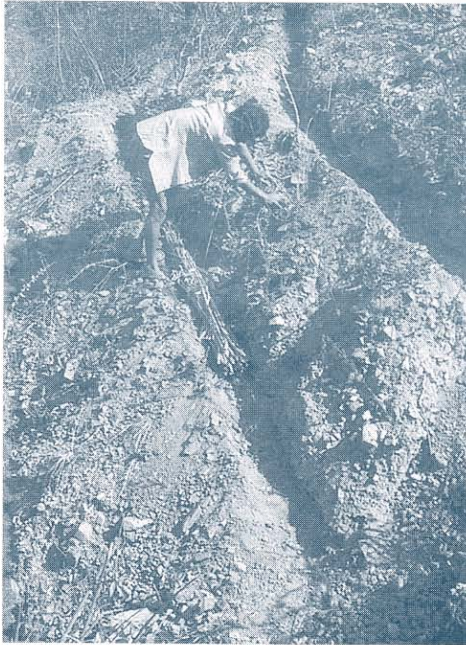
Fascines are effective on consolidated debris. They put out roots and shoots which develop into a strong line of vegetation, catching falling debris as well as armouring and reinforcing the slope
