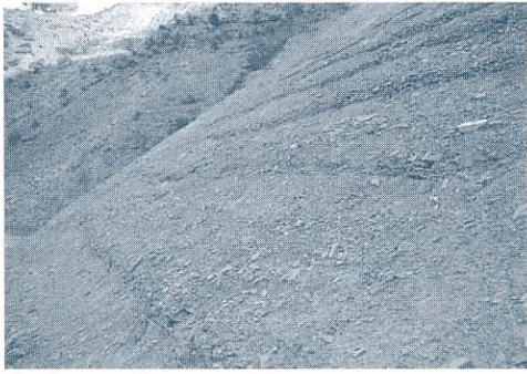
Completed wire bolster cylinders on a steep colluvial slope
