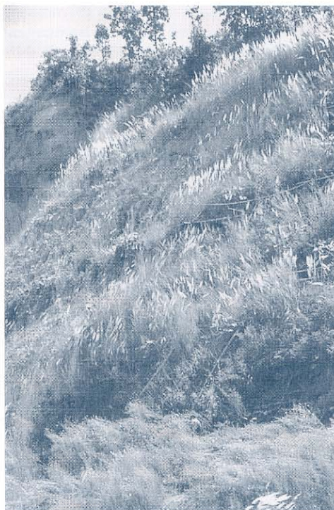
hydro-seeding can yield spectacular results for surface covering, but this example was estimated to cost about thirty times more than the manual method
