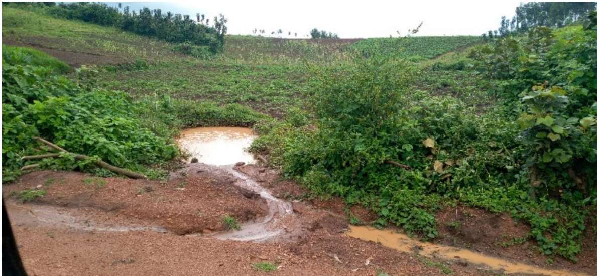
Figure 2-2 A small pond created near the road, this can flood the road on heavy showers
