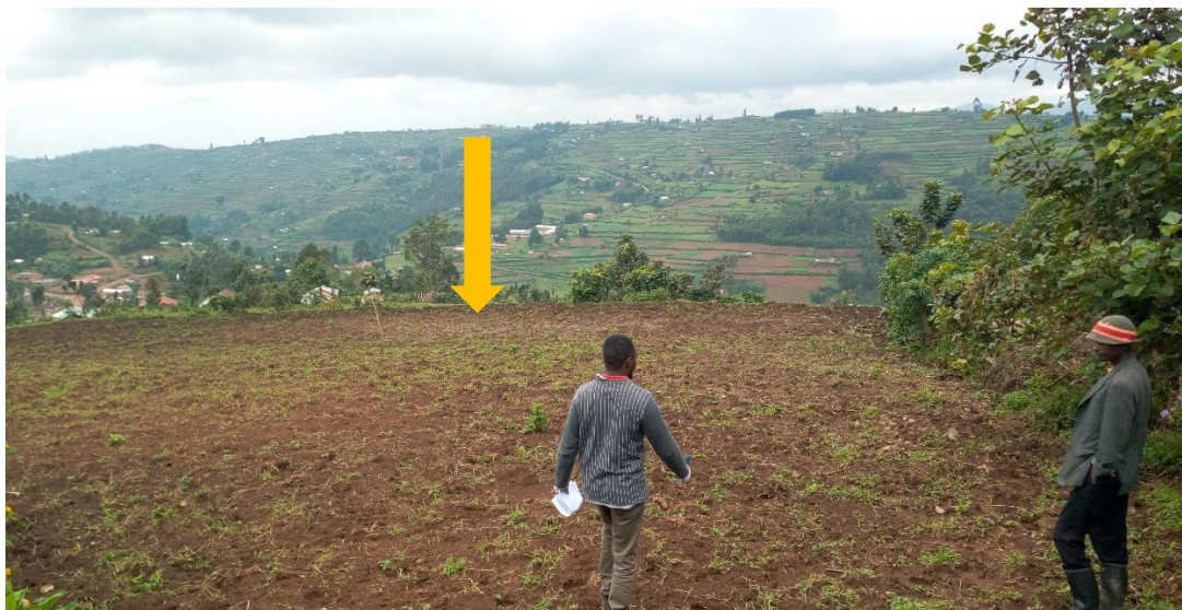
Figure 2-5 Shows field that gets flooded by water from culvert, see arrow
