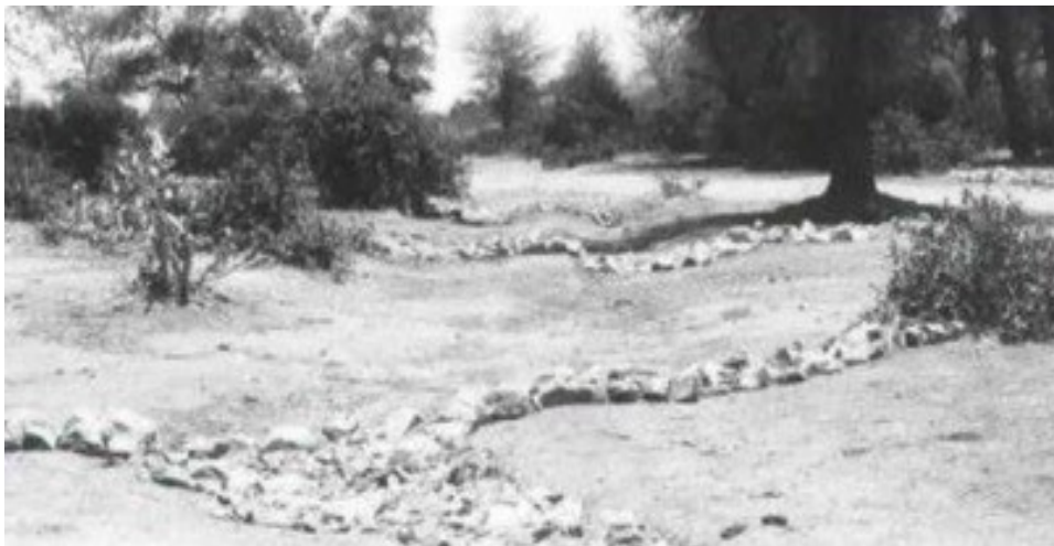
In slopy terrain: V-shape
