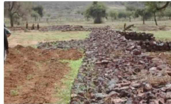
E: T-shaped rock bunds reinforce infiltration bund in erodible areas
