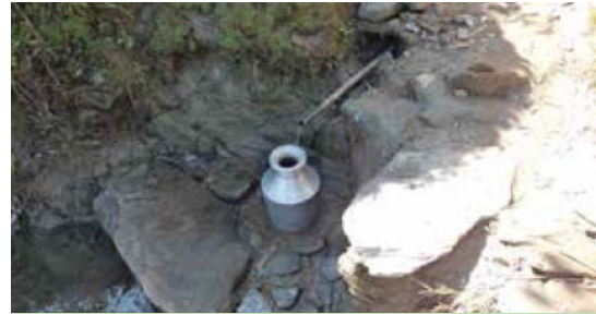
Polythene pipe conducting water from a dhara
