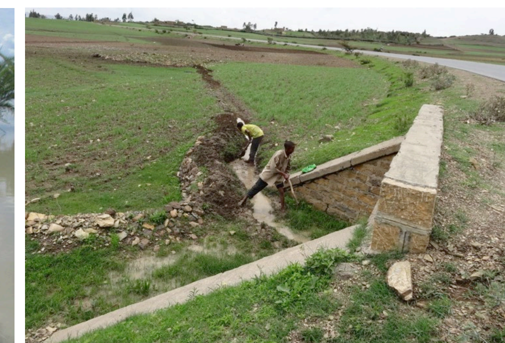
Water spreaders from culvert for supplemental irrigation
