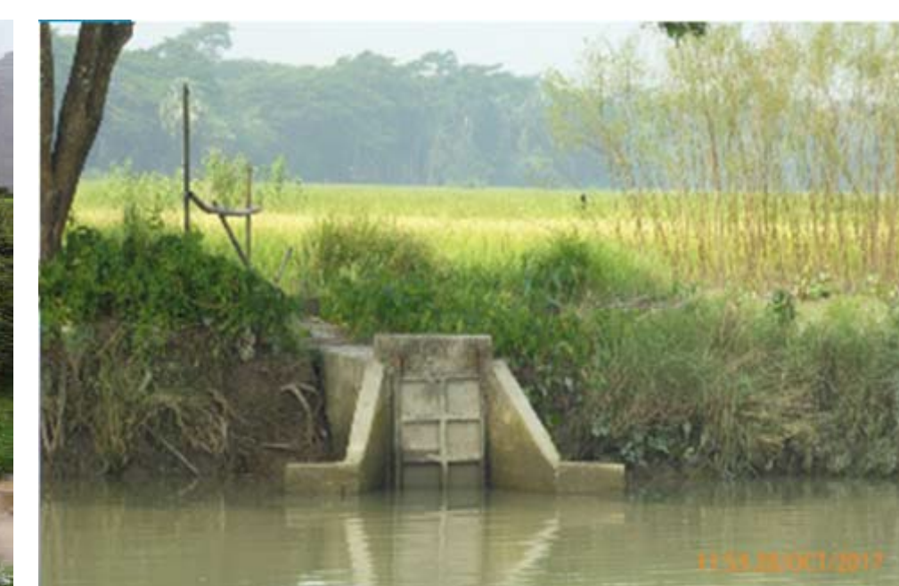
Flood Compartmentalization and gated culvert
