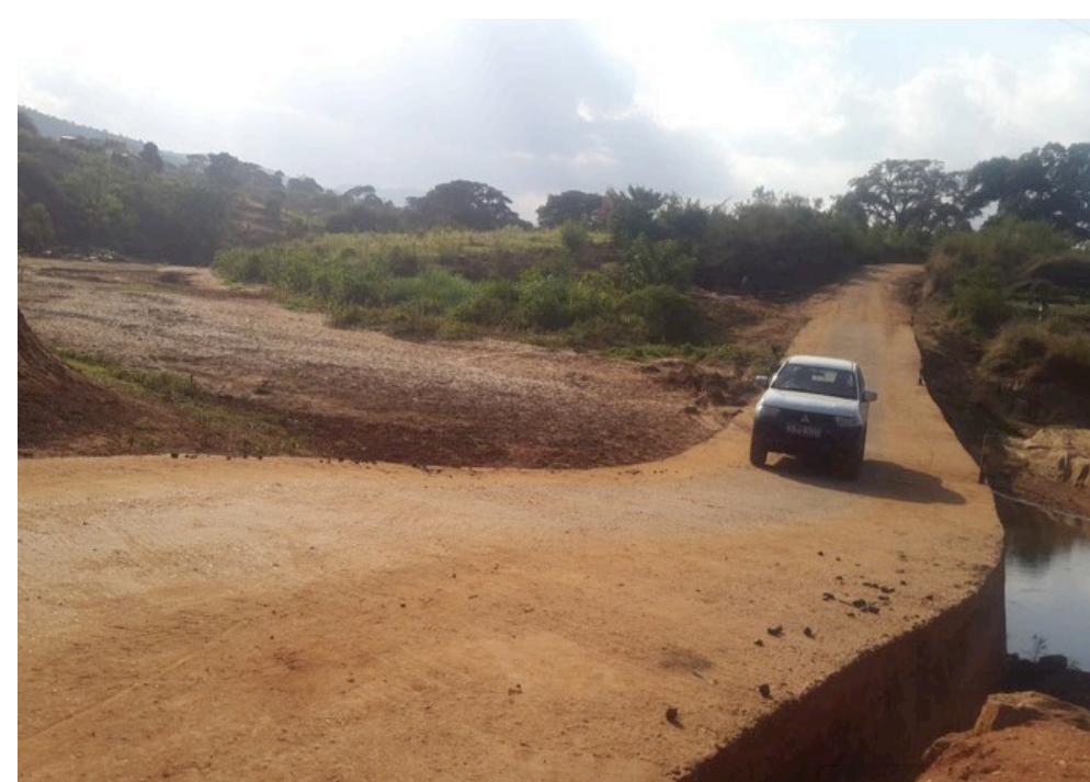
Road drift doubles up as sand dam for water retention
