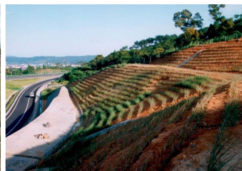
Bio-engineering protect the road-side slopes
