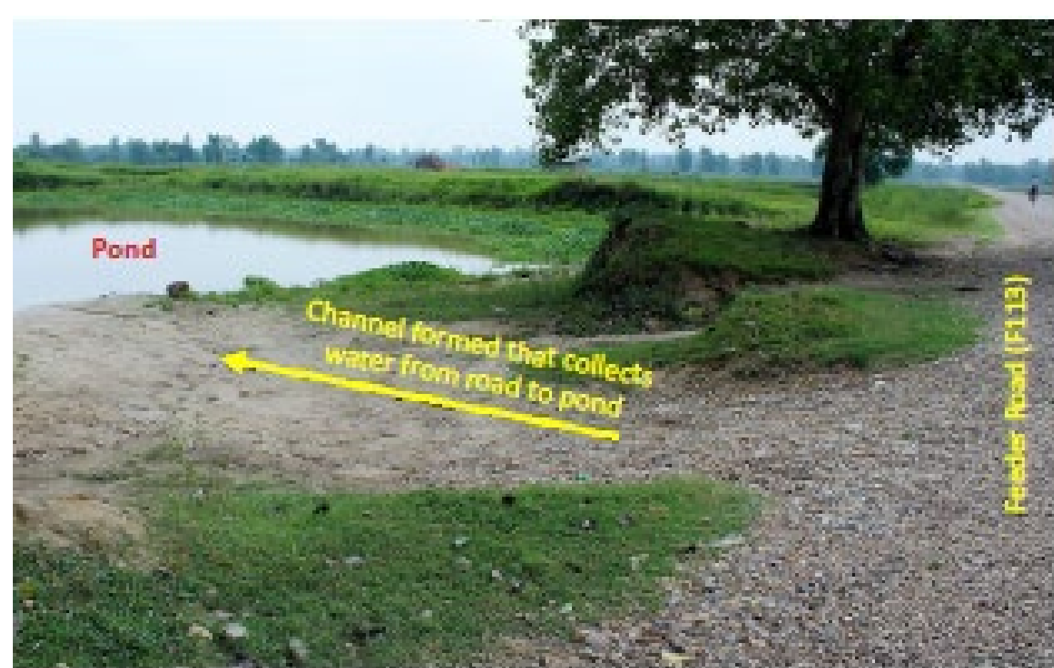
Road drift doubles up as sand dam for water retention
