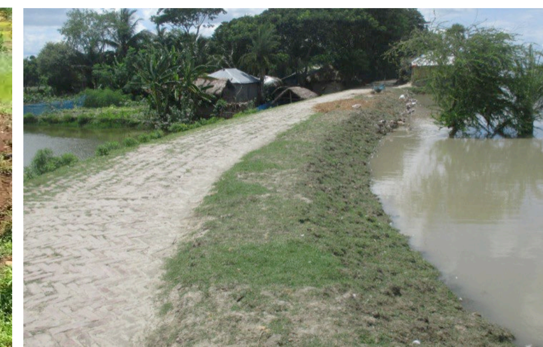
Roads serving as embankments in flood prone areas
