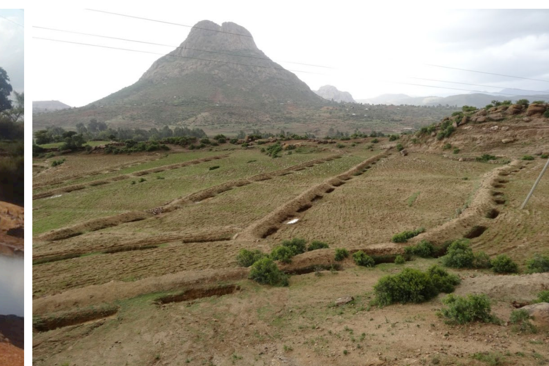
Roadside infiltration trenches in the large catchment
