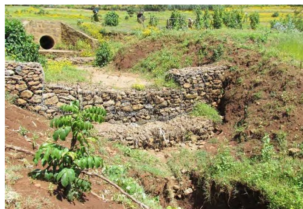
Gully plugging for recharge
