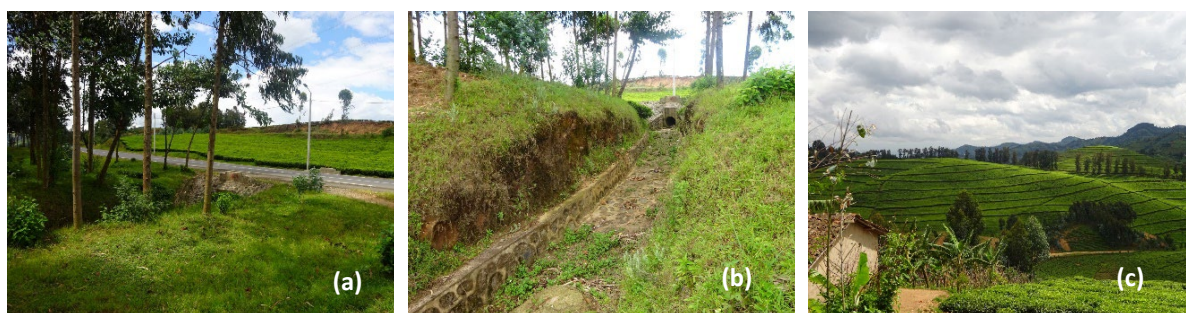
Figure 16: Masonry drains constructed at the culvert outlet to divert road runoff to tea plantations downstream of the road in Sebeya catchment (a) Road runoff collected from tarmac road, (b) Masonry water way constructed at culvert outlet, (c) Tea plantation benefiting of road runoff.
