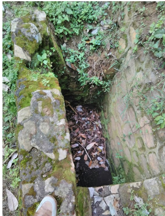
Figure 13: Culverts partially and fully clogged on feeder roads in Sebeya catchment.
