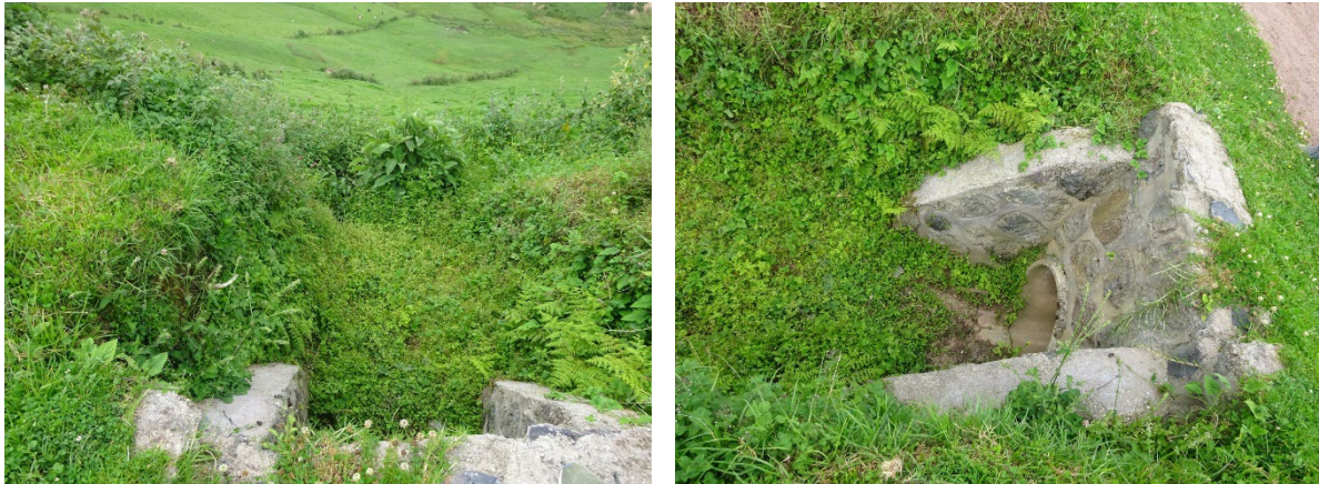
Figure 21: Grass vegetation at the culvert outlet protects the roadside environment from road-induced erosion.
