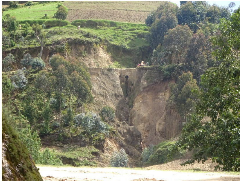
Figure 12: Erosion downstream of culvert in Sebeya catchment.
