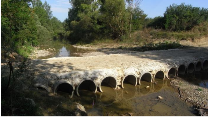
Vented drift that evacuates water and sand at crossing points
