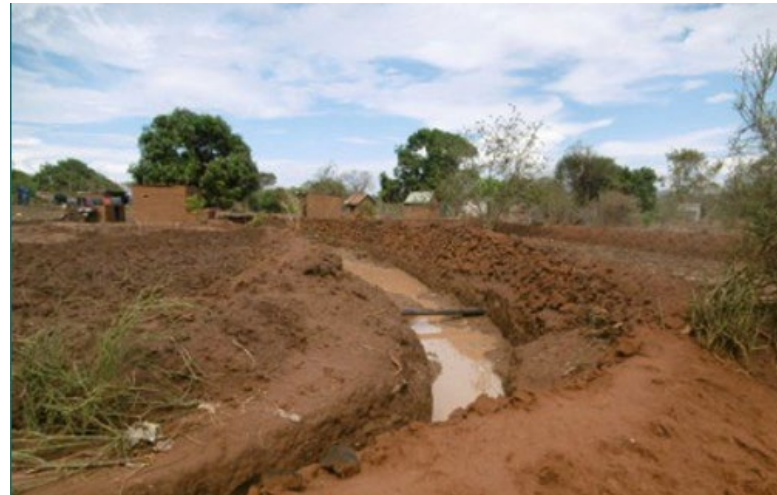
Feeding soil moisture with road drainage
