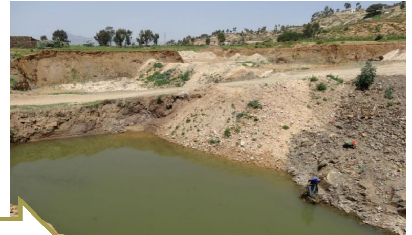
Converting borrow pits to store water from roadside drains and culverts
