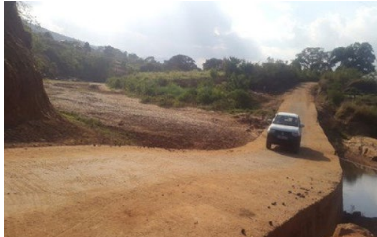
Retaining water with road drifts
