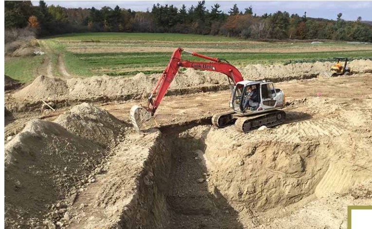
Converting borrow pits to store water from roadside drains and culverts
