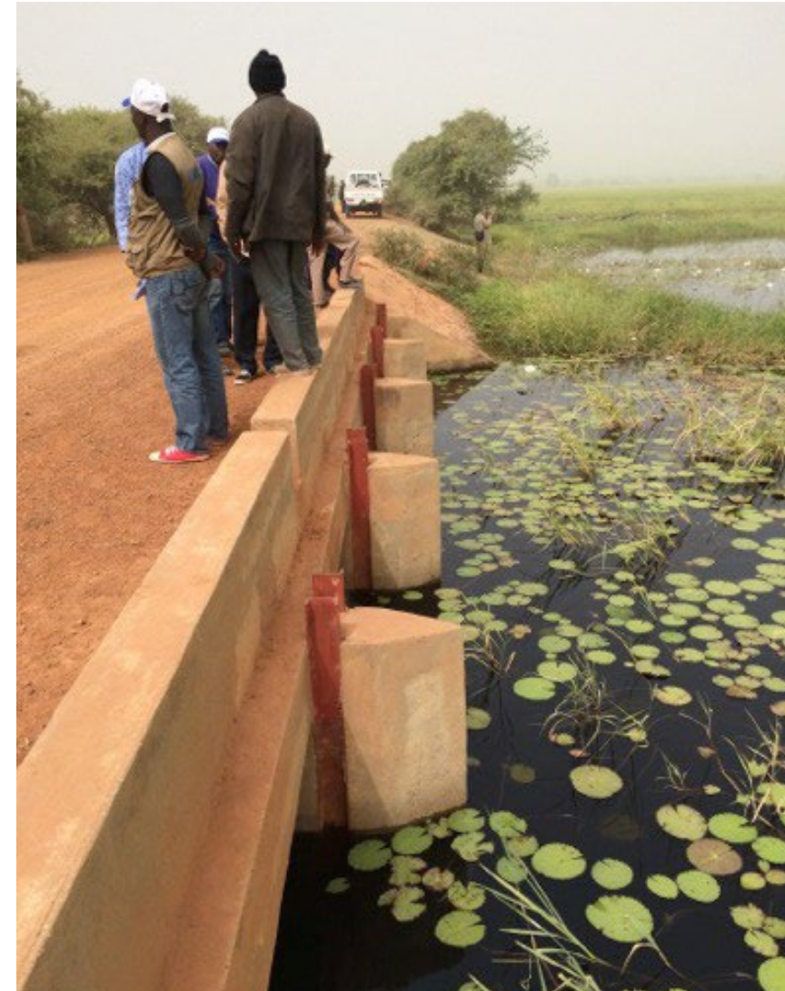
Road embankment creating storage reservoir
