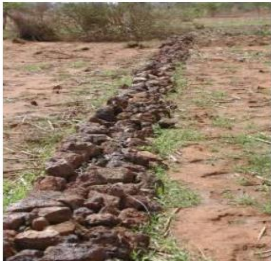
Stone bunds (embankment) along unpaved road to reduce erosion
