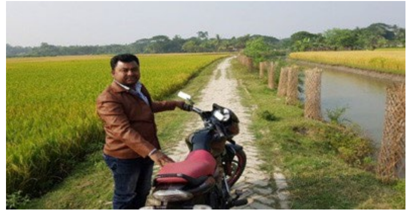
Road made from excavation of drainage canal
