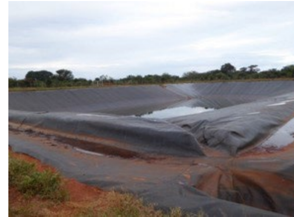
Converted lined borrow pit
