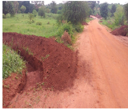
Road with Green Roads for water structures for road maintenance and farming.
