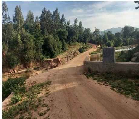
Non-vented road Drift as a road crossing & water storage structure.
