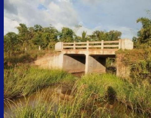
Using appropriate size culverts
