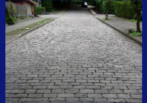
Pavers on streets through an urban area
