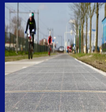
Energy generation with roads
