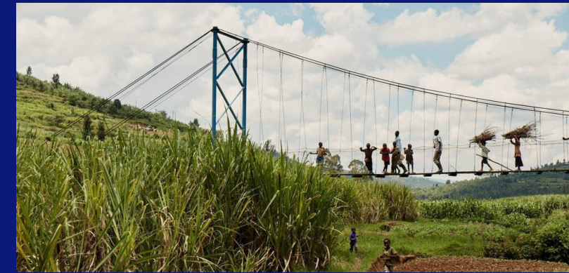
Trail bridge to ensure last mile access
