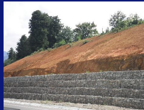
Stabilization of slopes
