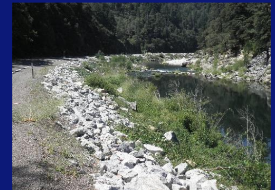
Streambank protection
