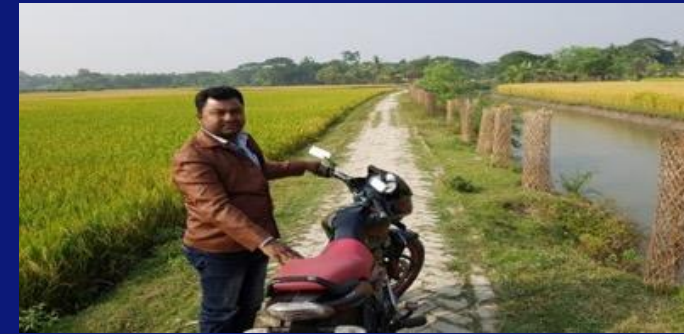
Road made from excavation of drainage canal
