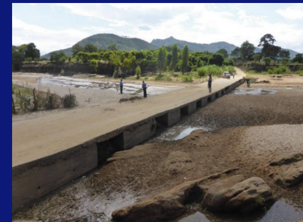
Road crossing doubling up as sand dam
