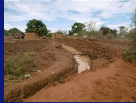
Field trench from road
