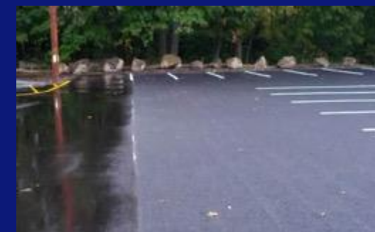
Porous pavement (right)
