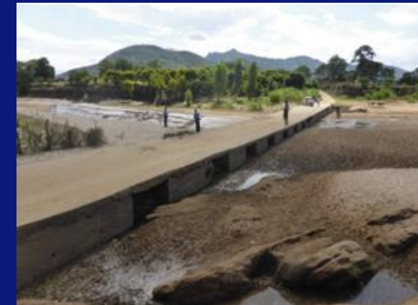
Road crossing stabilizing river course
