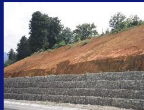
Stabilization of slopes
