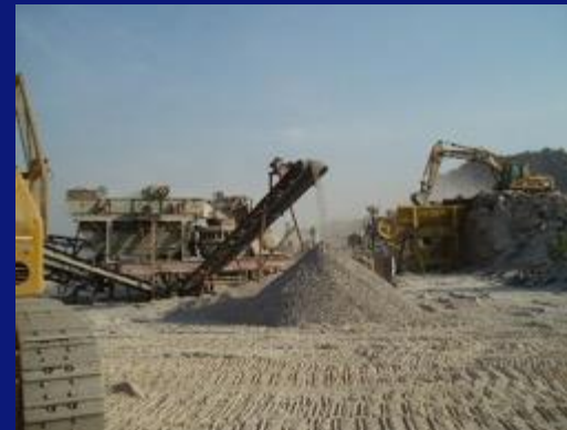
Local material processing
