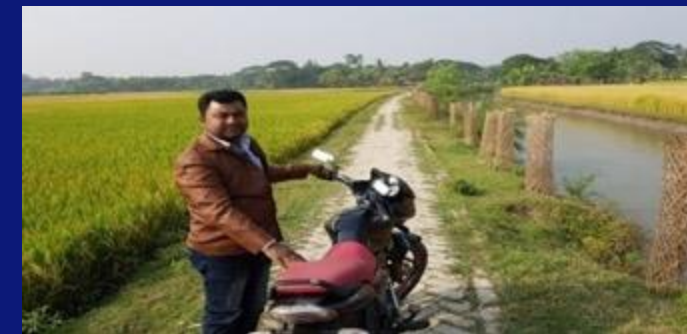
Road made from excavation of drainage canal
