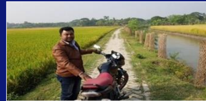
Road made from excavation of drainage canal
