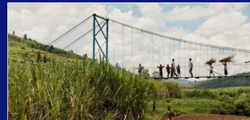
Trail bridge to ensure last mile access
