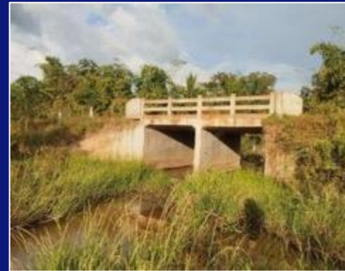
Using appropriate size culverts
