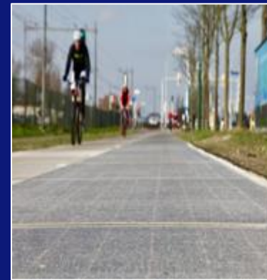
Energy generation with roads
