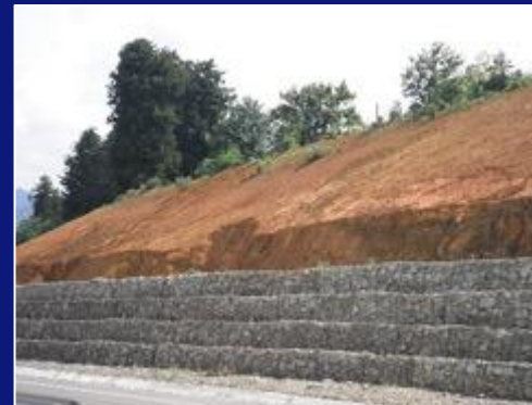
Stabilization of slopes
