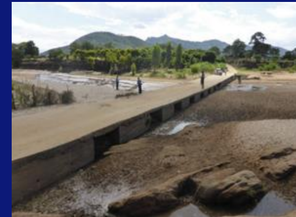
Road crossing stabilizing river course
