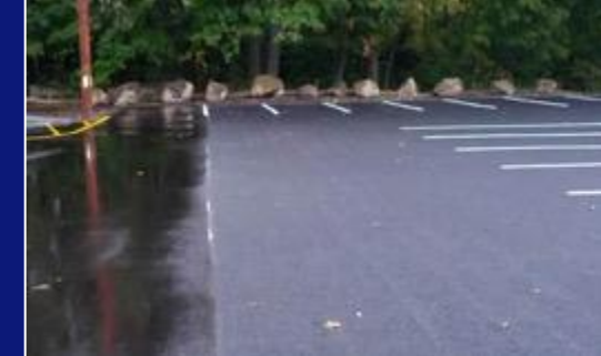
Porous pavement (right)
