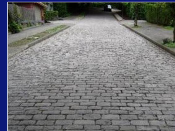
Pavers on streets through an urban area
