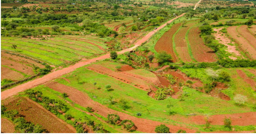
Road with cut-off drains and NBS Gully control
