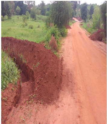
Cut-off drains/Mitre drains for runoff harvesting
