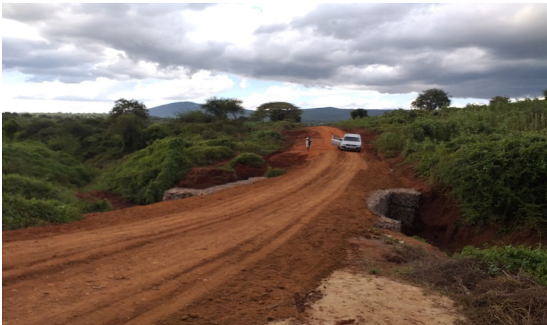
Deep gully –Gabions as protection works.
