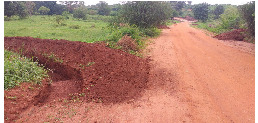
Road with Cut-off drains-Mud mitigation.
