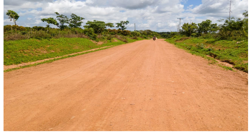
Green road with cut-off drains-Erosion mitigation.
