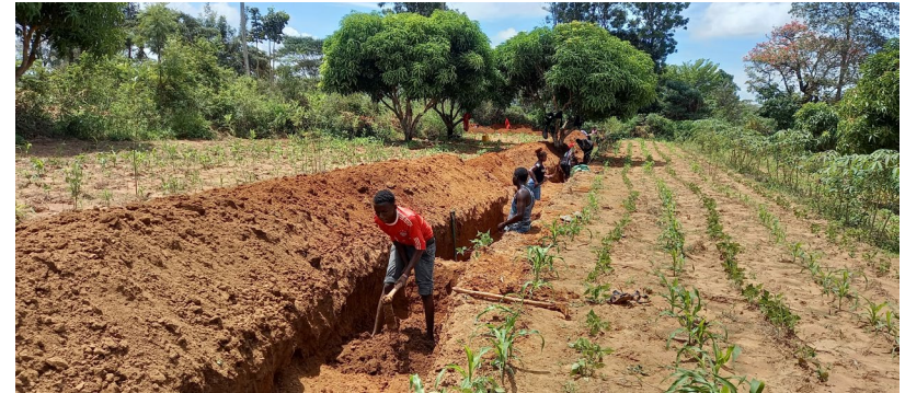
Engaging local communities in excavation of Green Roads for water structures-Cut-off drains
