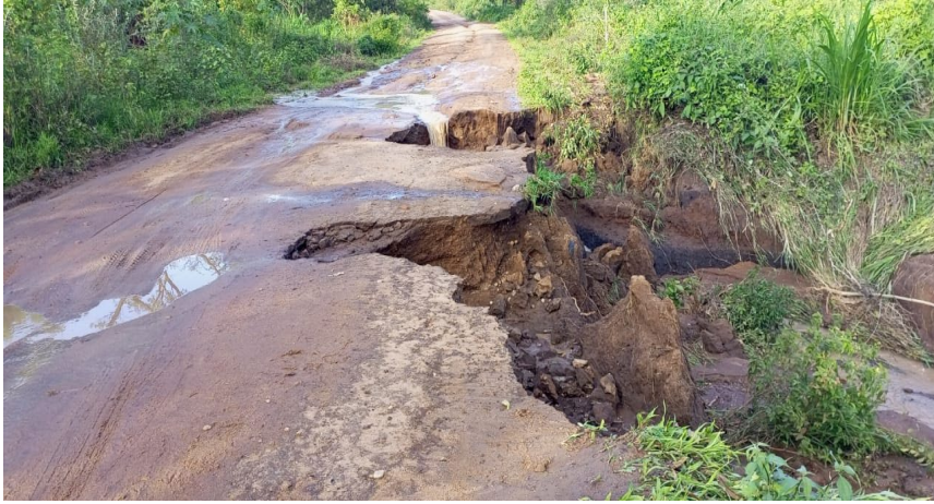
Eroded road section
