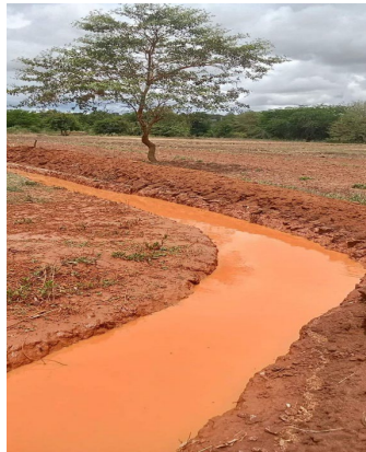
Cut-off drains/Mitre drains for runoff harvesting
