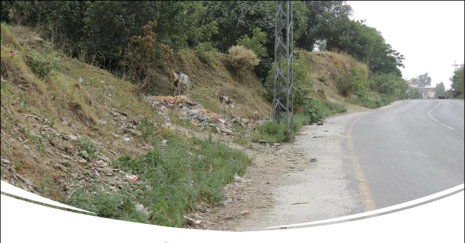
Lack of access control – blocking side drains
