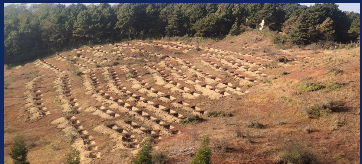
Spring shed improvement to enhance recharge
