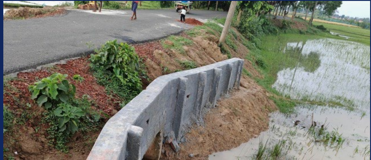
Retaining wall to be anchored (1/3) and backfilled
