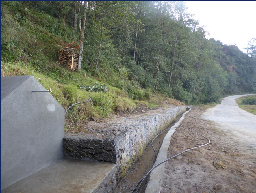
Roadside spring capture and protection
