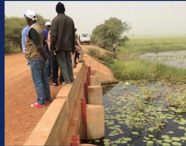
Water reservoir created with road embankment
