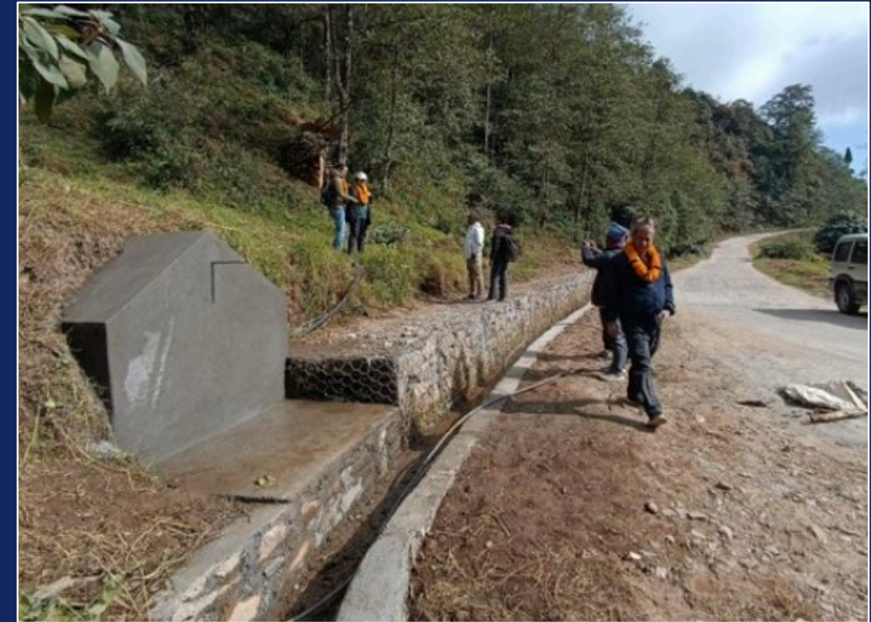
Roadside spring captured and developed
