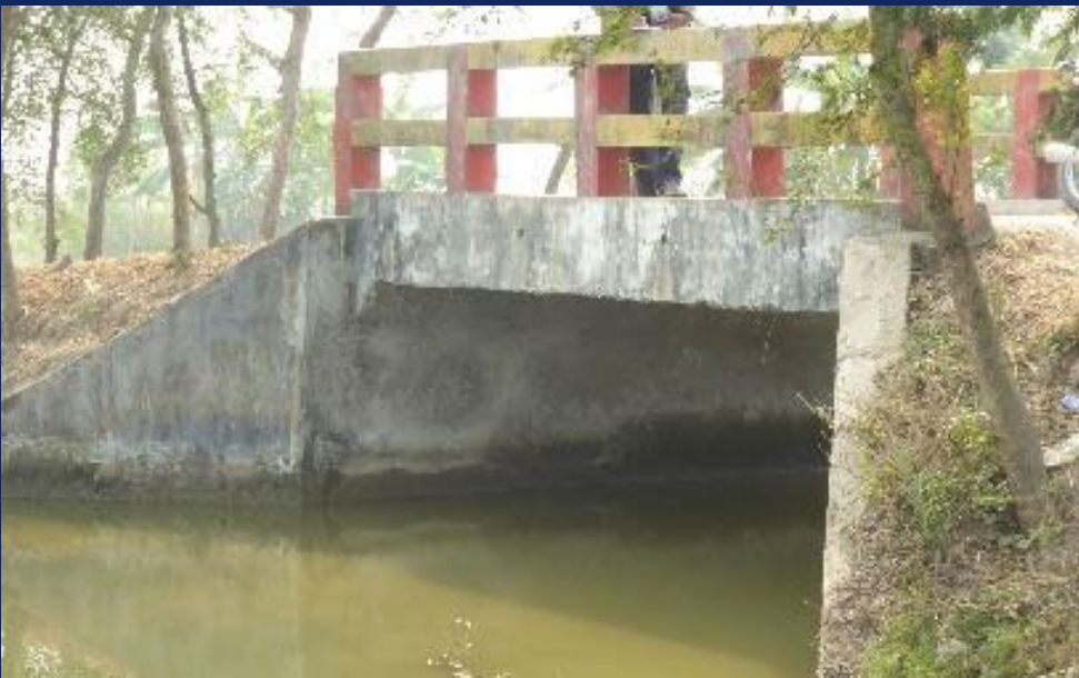
Sufficient cross drainage to avoid water logging
