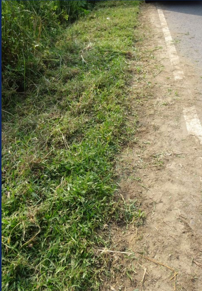
Grasses protecting side slope
