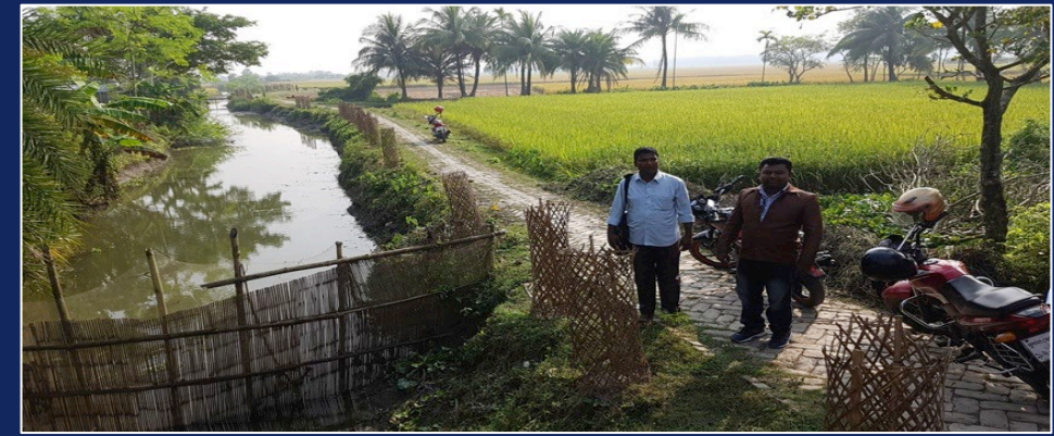
Road developed with excavated silt
