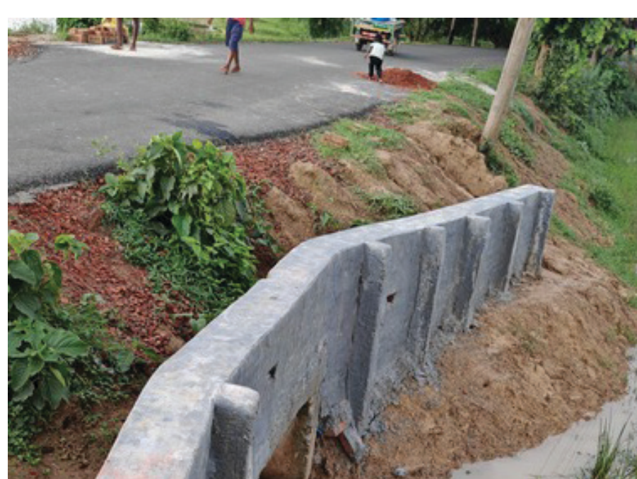
Retaining wall to be anchored (1/3) and backfilled
