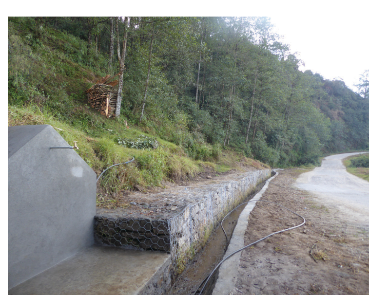
Roadside spring capture and protection
