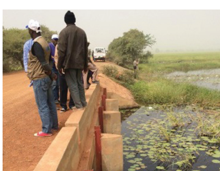
Water reservoir created with road embankment
