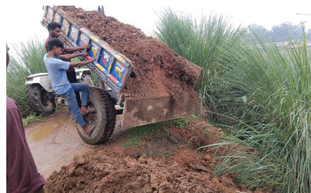
Damage to sideslope to be not just restored but be 'build back better'
