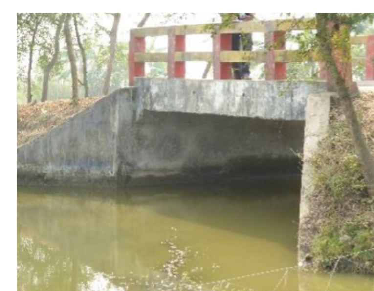
Sufficient cross drainage to avoid water logging
