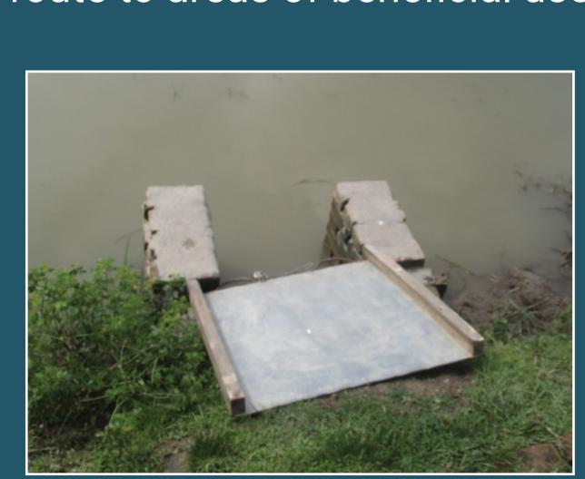
Gated culvert making it possible to control water levels in rice fields for optimum production
