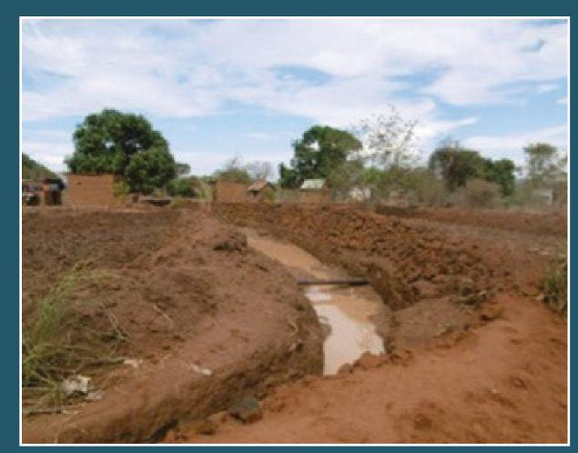
Road drainage water channelled into farm trench to irrigate root zones of the plants
