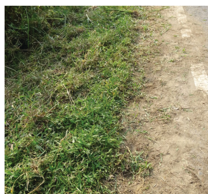
Grasses protecting side slope
