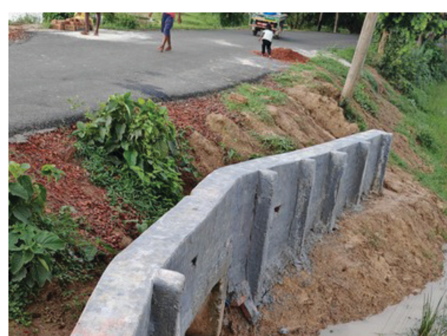
Retaining wall to be anchored (1/3) and backfilled
