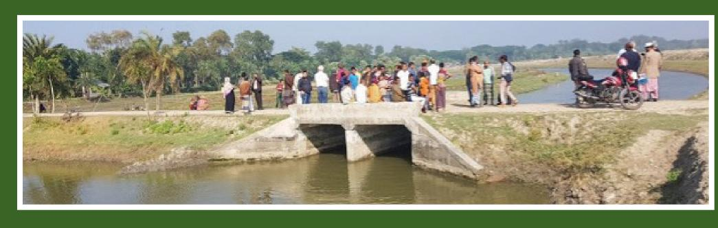
Bridge sill too high and bridge too narrow: causes water logging and silting up of the stream
