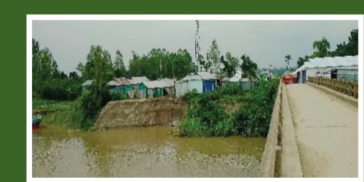
Bridge abutment and bridge approach vulnerable to erosion – need to solve with bio-engineering measures and armouring
