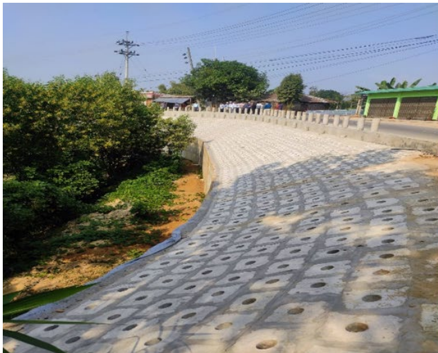
Figure 87 Roadside protection wall with hollow blocks, with geo-bags placed under the blocks.
