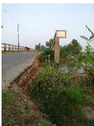
Figure 100 Scour / erosion / bridge. Photo taken on road assessment from Tarash to Singra.
