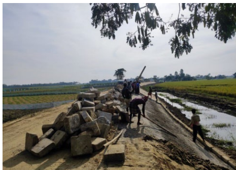
Figure 69 Block placing in the road slope to prevent erosion
