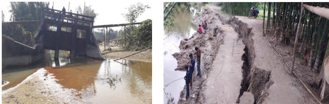
Figure 15 Due to shortage of cross drainage, water weakens the vulnerable section near the culvert and bridges, causing the roads to be undermined.
