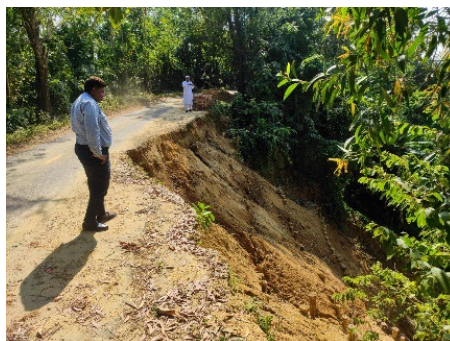
Figure 75 Road erosion due to runoff water
