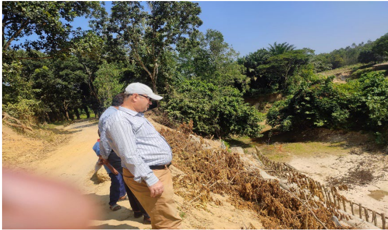
Figure 86 A site of the hilly Bandarban District in Sadar Upazila. On the right side of the road, there is ballah pilting for slope protection. On the left side of the road, there is a slope from which water flows down during monsoon season. Bioengineering is a promising approach on this site.
