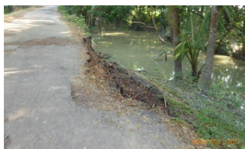
Figure 9 Damage to road carpeting
