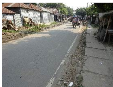
Figure 91 No drainage facilities. Photo taken on road assessment from Tarash to Singra.
