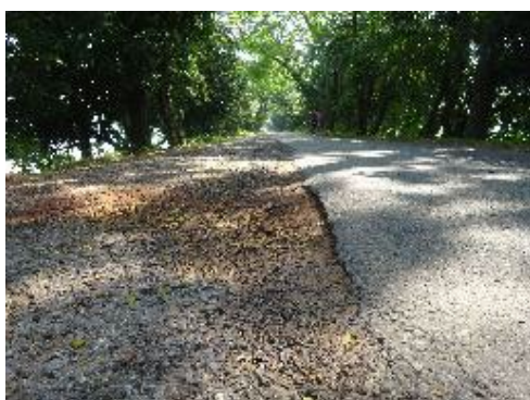
Figure 110 Left in frame: poor construction and damaged, right in frame: good construction and no damage. Photo taken at road assessment from Singra towards Atrai / Naogoan.
