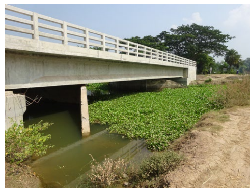
Figure 18 Bridge being reconstructed with more drainage potential
