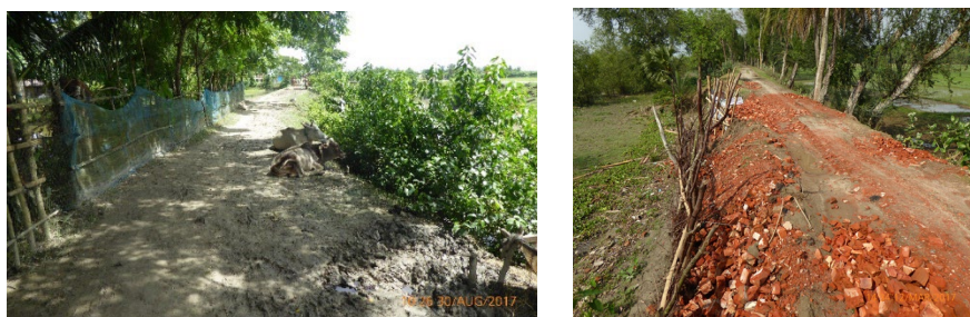
Figure 4 Damage to road (left) and inadequate construction material (right)
