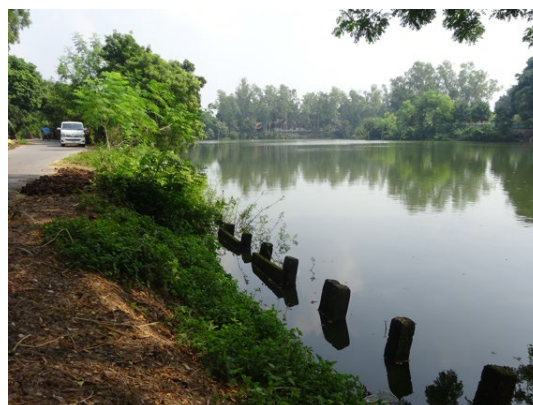
Figure 10 Shoulder wall to keep shoulder in place (partly successful)
