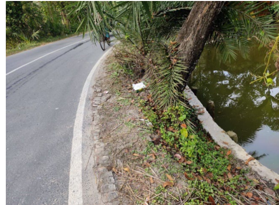
Figure 44 Narrow shoulder in bend
