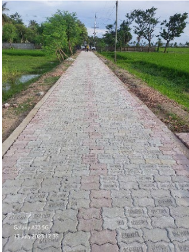
Figure 43 Uni-block road without bituminous black top/ 2-20%
