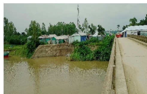
Figure 17 Protection of river banks and abutment of bridge using vegetative measures
