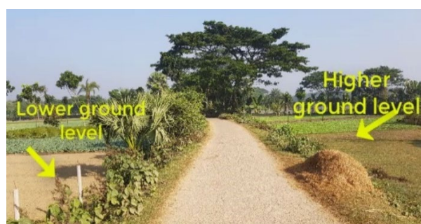
Figure 23 Impact of road on ground level; using roads as a sediment trap
