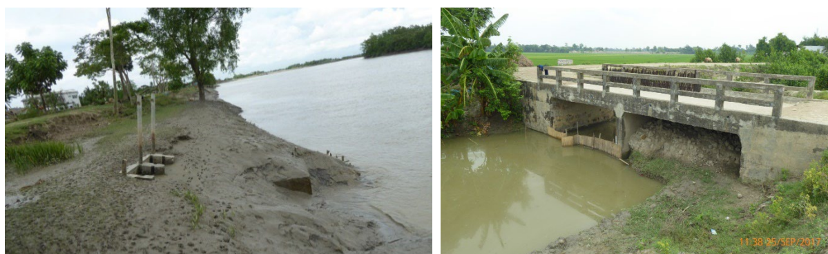
Figure 7 Left: Silted sluice, Right: Silted bridge
