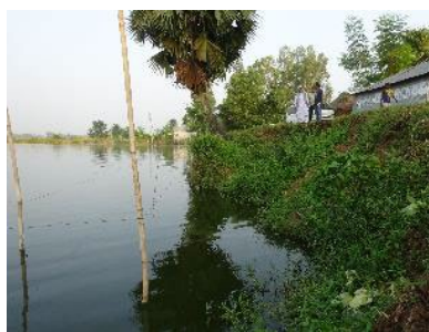
Figure 96 Eroded shoulder with pond very close to road. Photo taken on road assessment from Tarash to Singra
