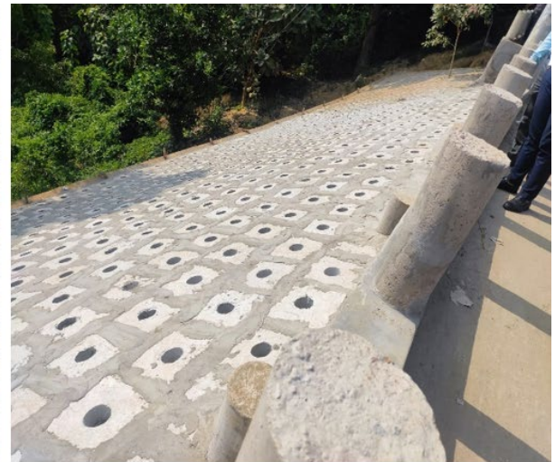
Figure 87 Roadside protection wall with hollow blocks, with geo-bags placed under the blocks.
