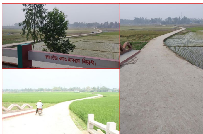
Figure 29 Submersible roads in Singra Municipality, Bangladesh ( https://singramunicipality.gov.bd/wp-content/uploads/2023/06/Submersible-road.pdf )
