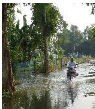
Figure 112 Water quickly flowing over road, eroding road and shoulders
