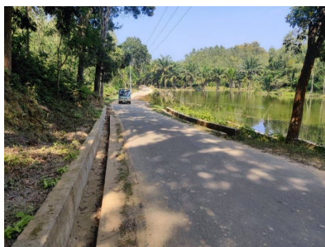
Figure 77 Drain (left side) with potential to be used for water storage
