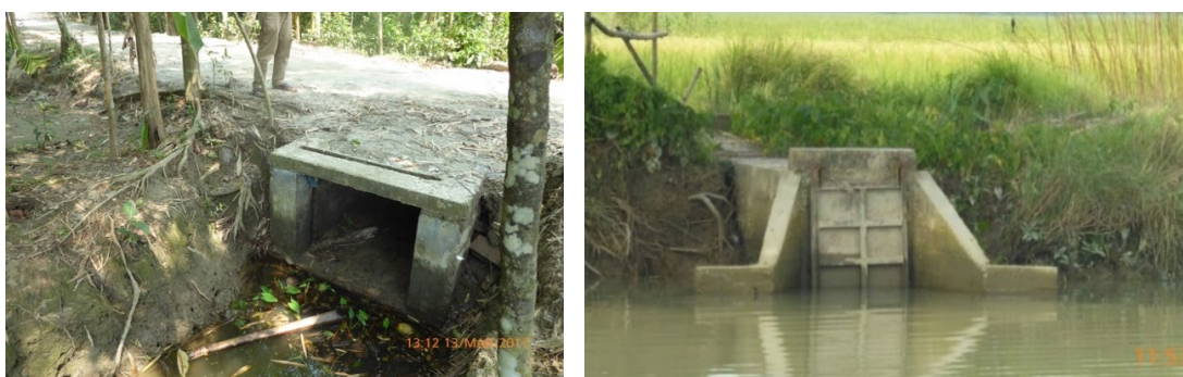
Figure 22 Left: Box culvert with slot for gate, Right: Gated culvert
