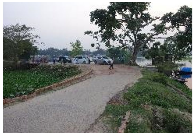
Figure 117 Road assessment near Atrai Upazila, where too small sluiceways cause road to overflow and damage roads. On this roads, interestingly, now a lot of young trees seem to have been planted.
