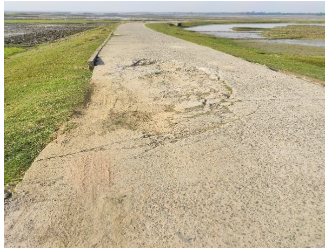
Figure 52 Road damage by tidal movements
