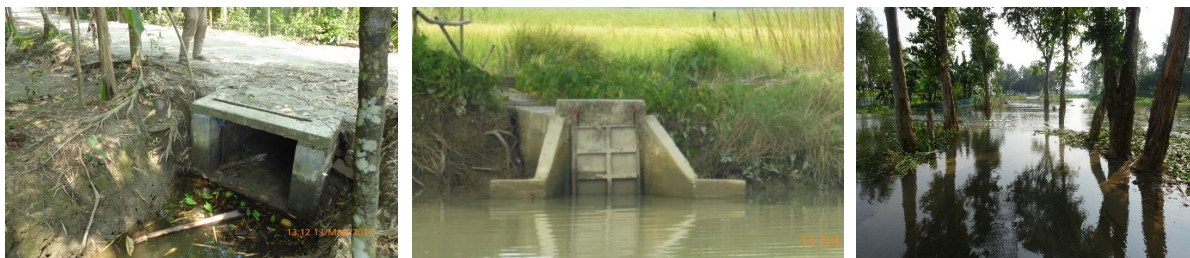
Figure 16 Left: Box culvert with slot for gate, Middle: Gated culvert, Right: Causeway
