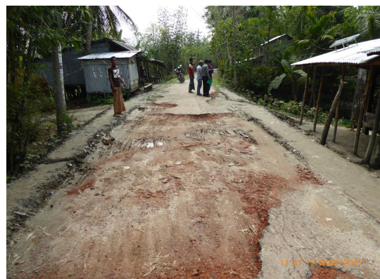
Figure 6 Inadequate carpeting
