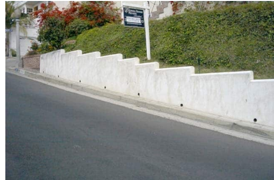
Figure 32 Weepholes provided at the bottom of a retaining wall ( https://civildigital.com/weep-holes-civil-engineering-structures-retaining-walls/weepholes/ )
