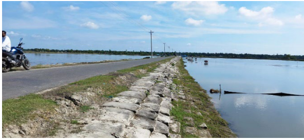
Figure 42 Road in coastal zone with side slope protection but no to limited vegetation
