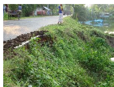
Figure 95 Eroded shoulder. Photo taken on road assessment from Tarash to Singra.
