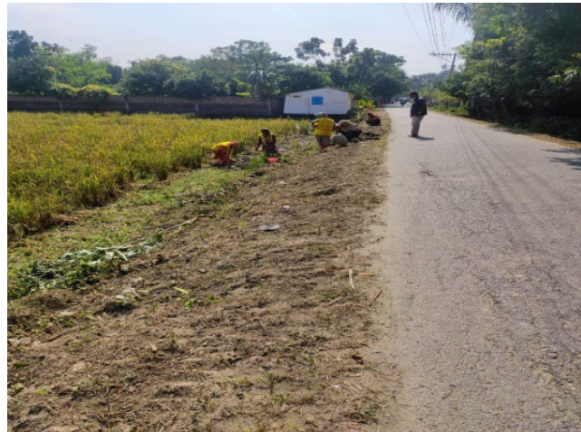
Figure 49 LCS cleaning the road shoulder
