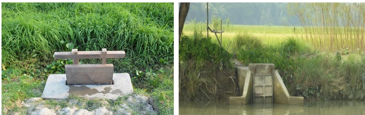
Figure 48 - Left: Engineered gated culvert in rice growing area, Right: Gated culvert discharging in local canal/ drain
