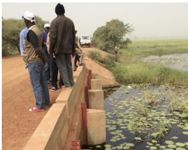
Figure 33 - Water reservoir created with road embankment
