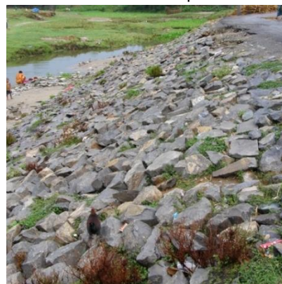
Embankment protection using riprap
