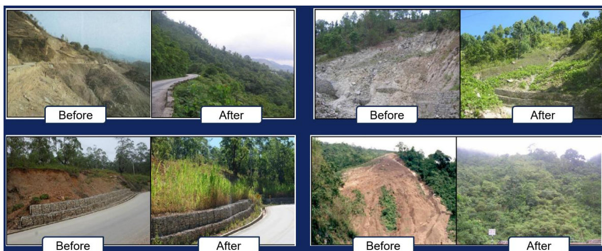
Figure 66 - Before and after images from bio-engineering
