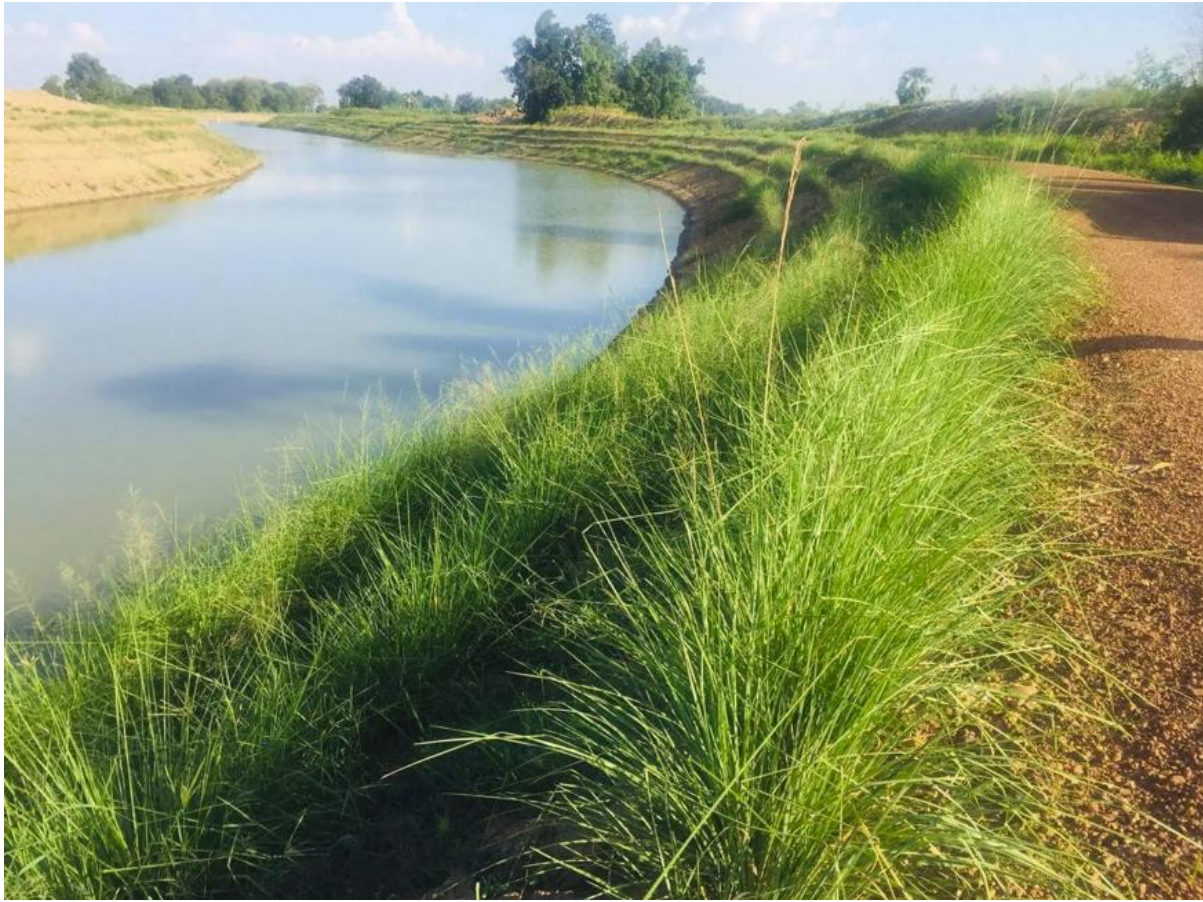
Figure 65 - Bio-engineering on road embankment
