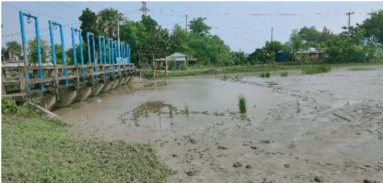
Figure 11- Bridge disturbing bed load of tidal river
