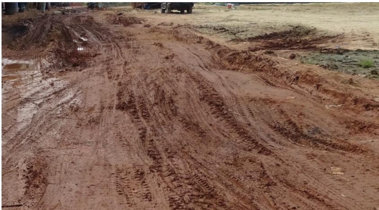
Figure 59- Water management measures and adequate maintenance are essential to ensure longevity of unpaved roads
