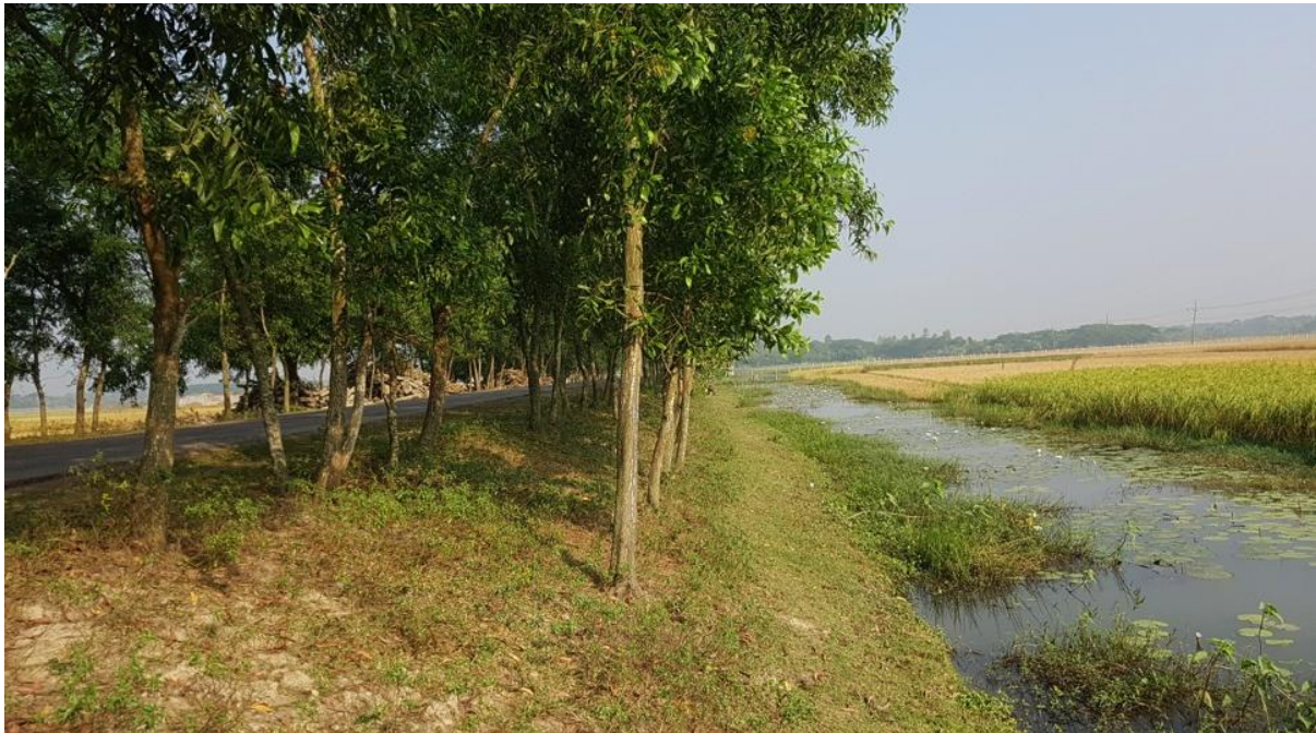
Figure 39 - Road embankment borrow trench cum multipurpose drain (notice distance from embankment may be increased)
