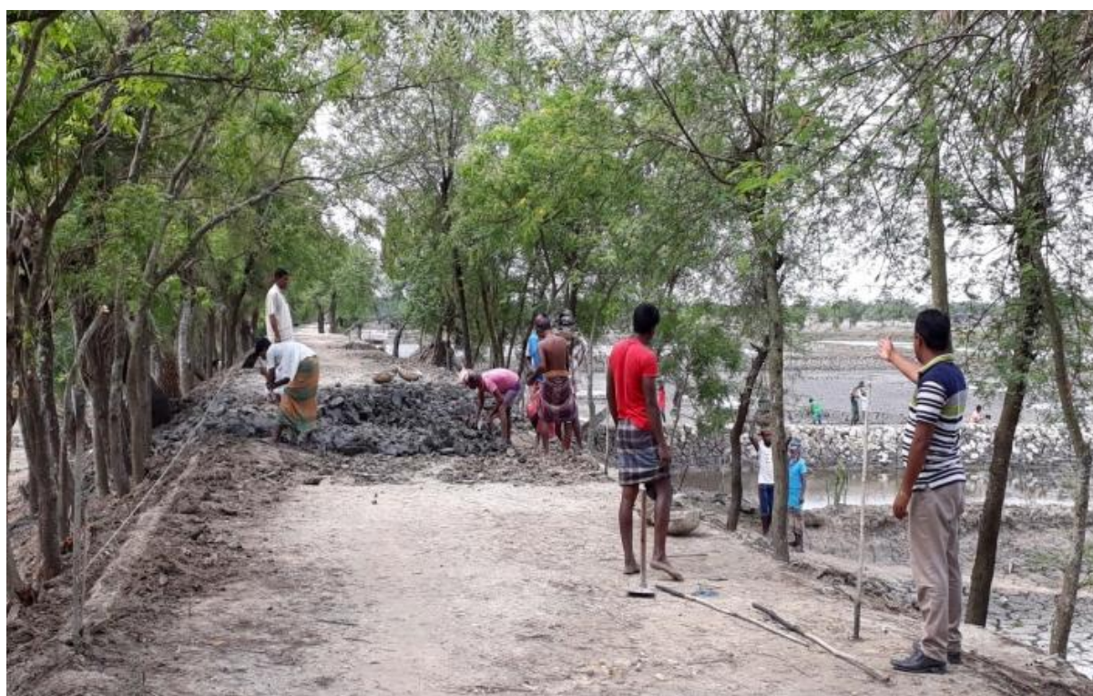
Figure 39 - During: Re-sectioning work of the embankment
