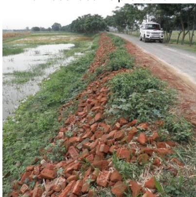
Embankment protection with brick armor
