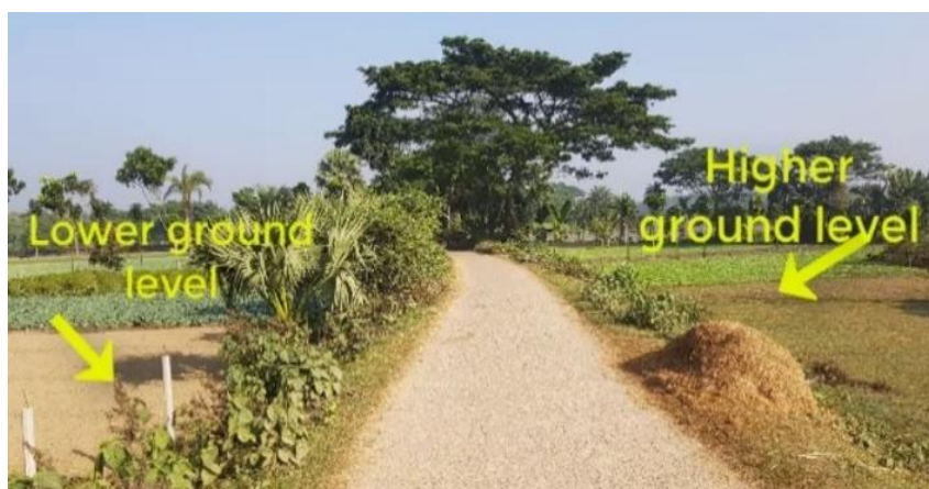
Figure 14 - Impact of road on ground level; using roads as a sediment trap
