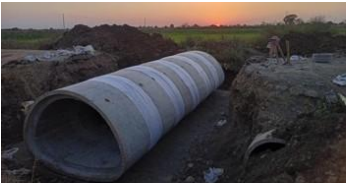
Figure 34 - Arched culvert for easier passage of fish and other creatures
