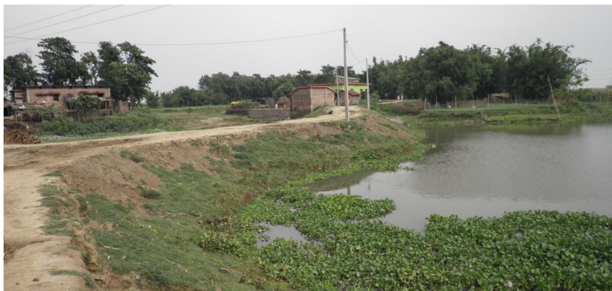
Figure 42 - Road embankment (tragically) blocking drainage (photo G. Keller)
