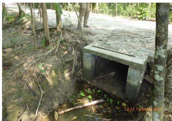
Figure 13 - Left: Box culvert with slot for gate, Right: Gated culvert
