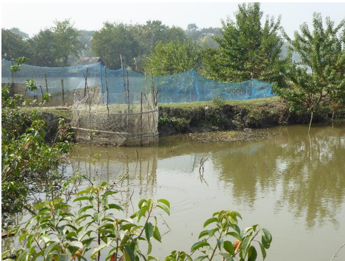
Figure 43 - Locally constructed embankment footpath with no cross drainage, causing drainage congestion – this may have to be corrected by retrofitting culverts or pipes
