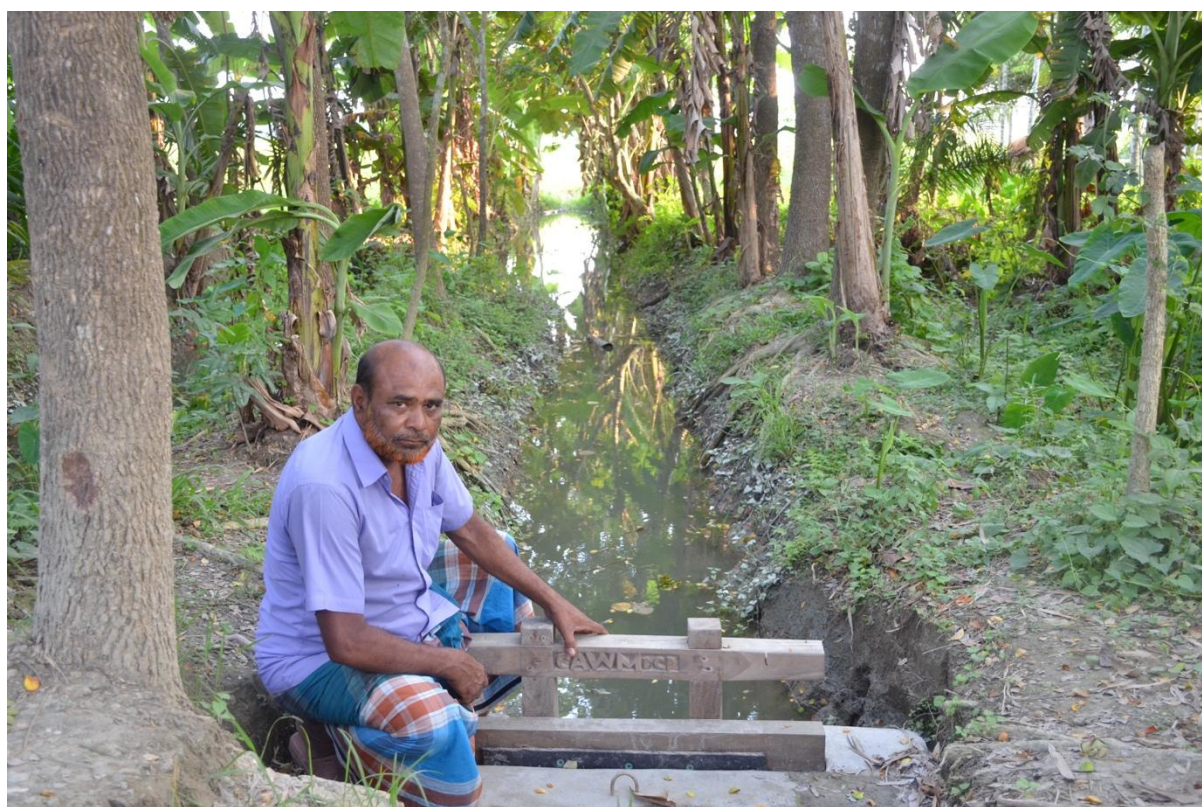
Figure 41 - Gated culvert to control water levels in rice fields
