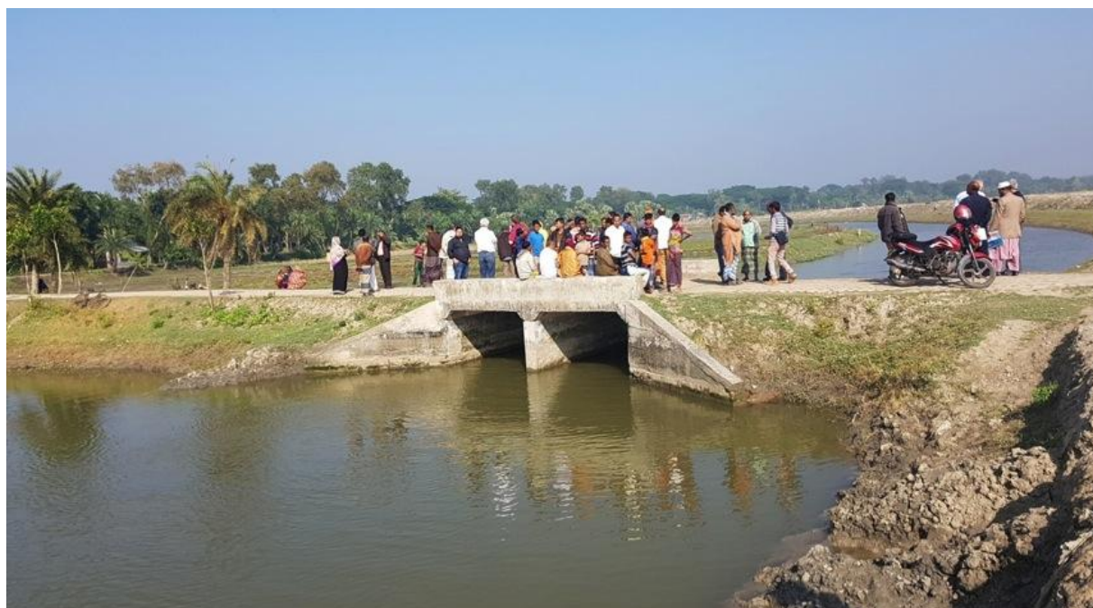
Figure 53 - Bridge causing congestions – natural stream restricted and bed sill too high
