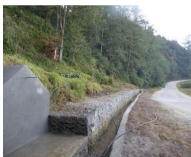
Figure 24- Left: Roadside spring capture and protection in Nepal, Right: Spring shed improvement to enhance recharge in Nepal
