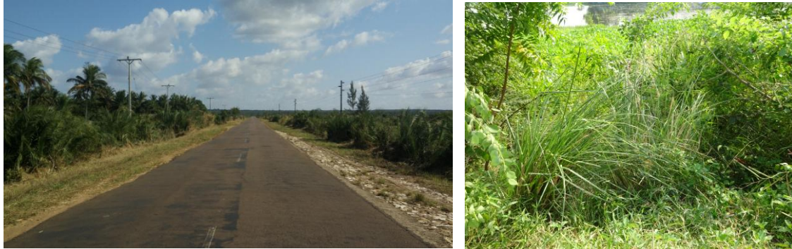
Figure 35 - Left: Overflow area with armouring and vegetative protection, Right: Vetiver grass as slope stabilizer
