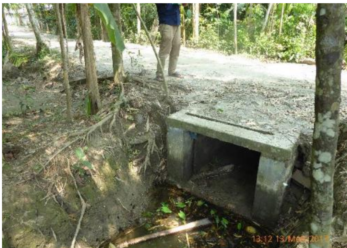
Figure 57 - Culvert with slot for temporary gate - this is very useful for water level control in the adjacent fields and is practice to be encouraged
