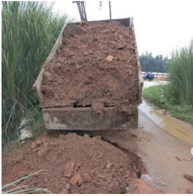
Backfilling and compaction (building back better)
