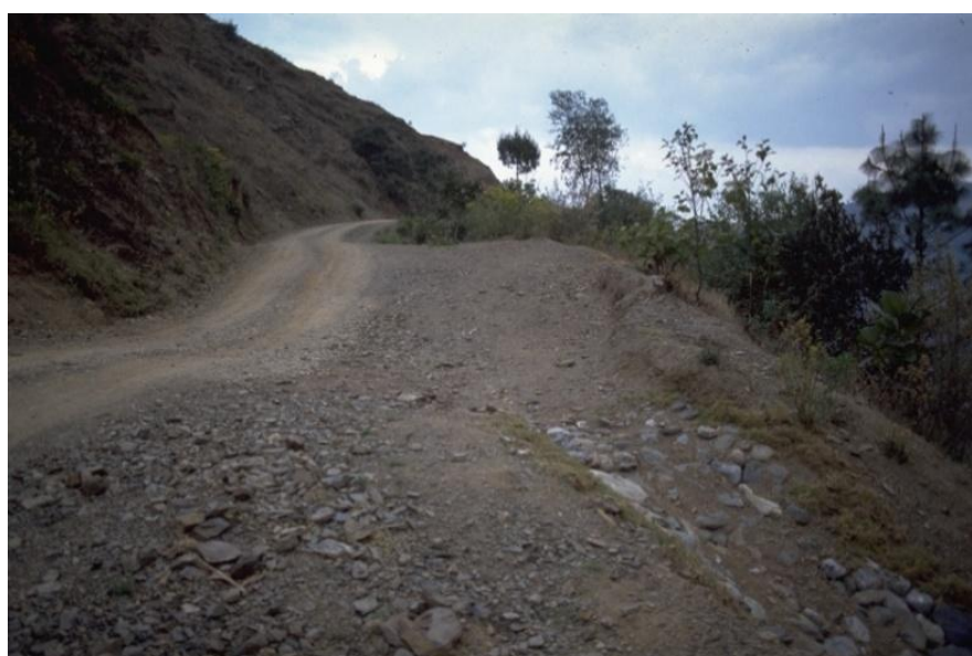
Figure 61 - Rolling dip in hilly area (photo G. Keller)
