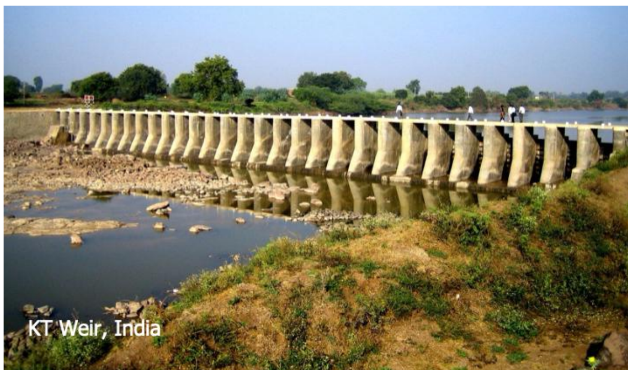
Figure 54 - Bandara-cum-bridge to retain groundwater
