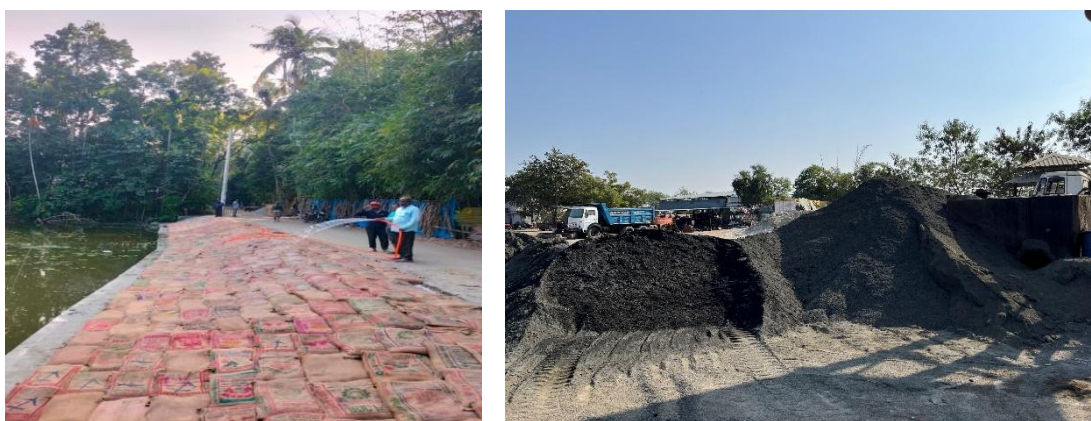
Figure 30- Left: Using porous pavement for water percolation, Right: Responsible sourcing: use manufactured sand instead of sand from vulnerable rivers
