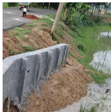
Retaining wall with proper backfilling
