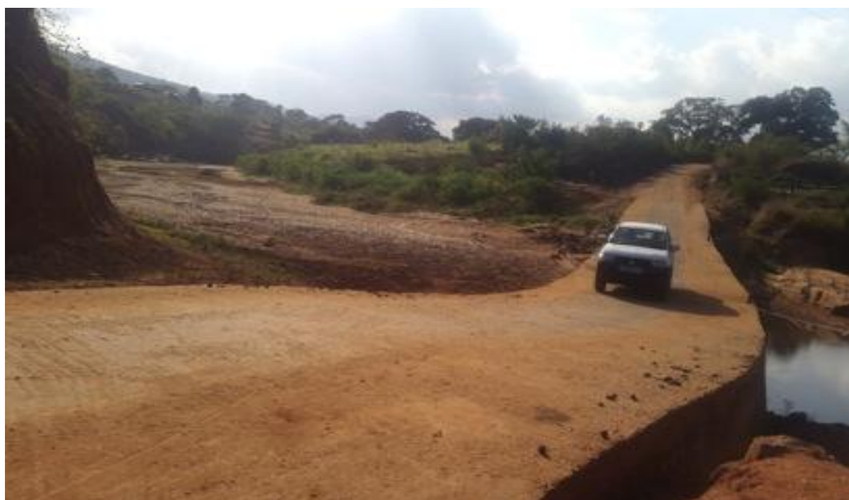
Figure 55 - Non-vented drift acting as sand dam
