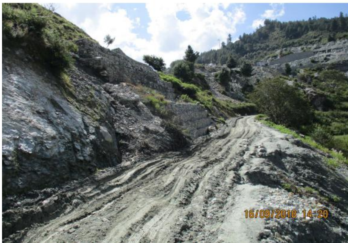
Figure 63 - Road damaged because of uncontrolled spring seepage
