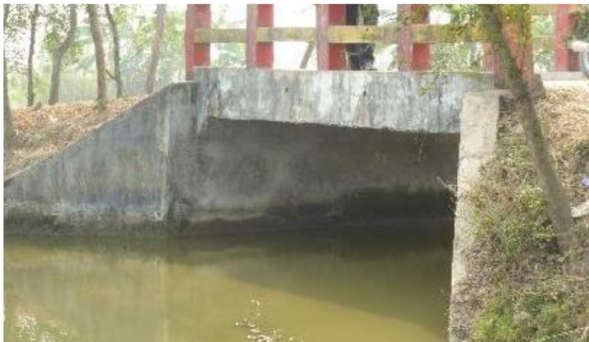
Figure 18 - Sufficient cross drainage to avoid water logging
