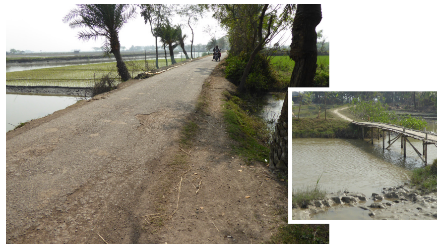
Figure 7: Main pucca Union Road cuts the Shaka Bai khal. Connectivity shall be restored by providing a large culvert on this road (left). A bridge is needed near Baloiyakhi Sluice. People use a bamboo bridge to transport goods (right).
