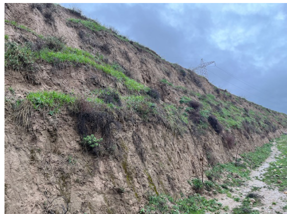
Pioneer plants on untreated slope – potential for use in bioengineering
