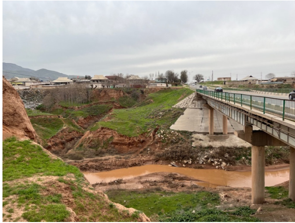
Riverbank erosion around bridge
