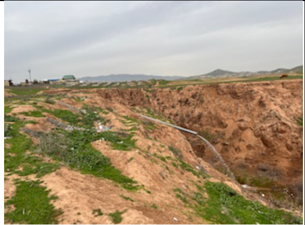
Massive bank erosion caused by uncontrolled outlet of land drain
