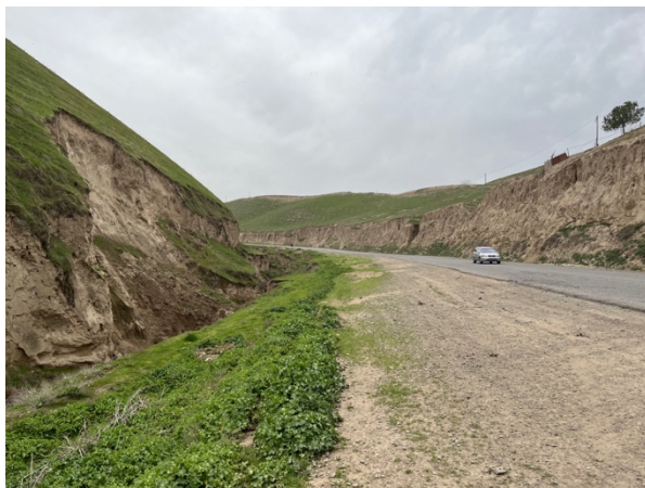
Weak side slopes along last road section
