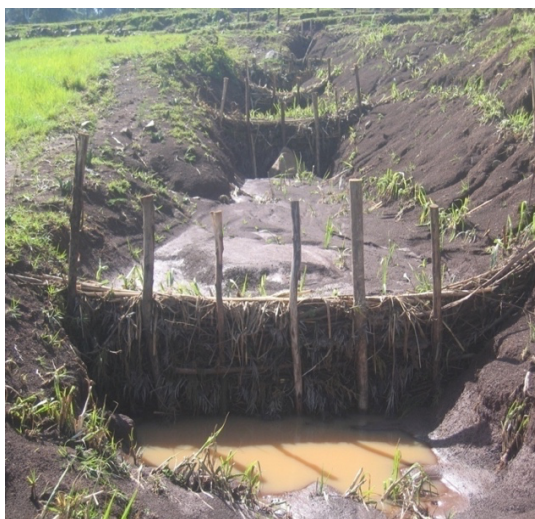
Gully plugging with vegetative screens.
