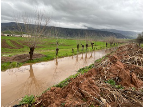
Drainage congestion in upper section of proposed road
